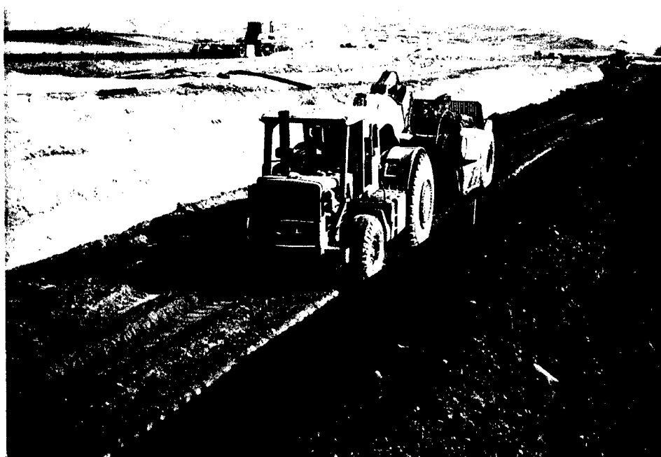
Photo 16 Cat 660 scraper dumping fill in the inspection trench. 15 Oct. 1990
