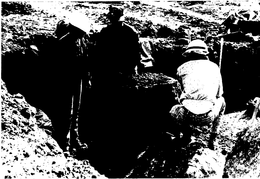
Photo 21 Early stages of carving undisturbed sample for record sample program. 3 Dec 1990
