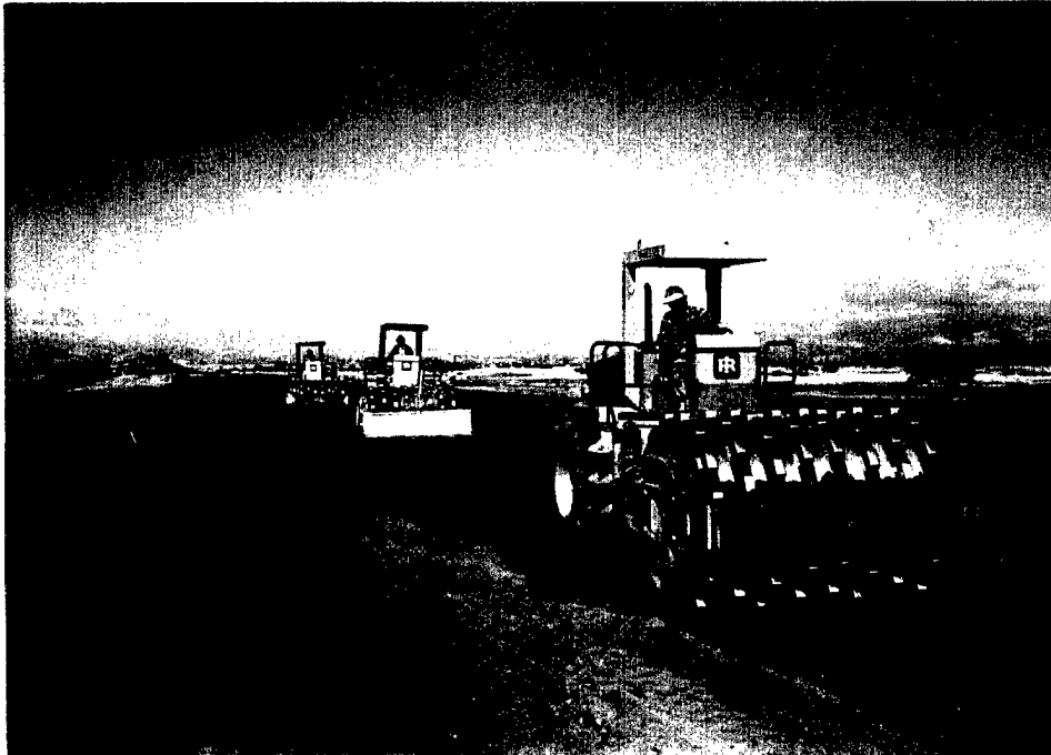
Photo 19 Dynapac and Ingersoll Rand rollers compacting the embankment. 15 Oct. 1990
