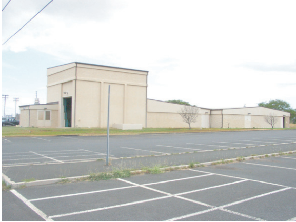
Bldg. 1874 (fire safety props to be installed in parking lot area)
