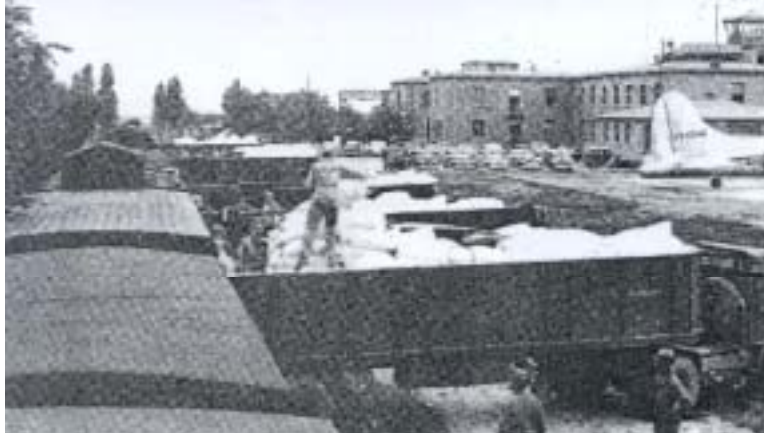
Figure 4 Loading Operations From Rail to 10-ton Truck
