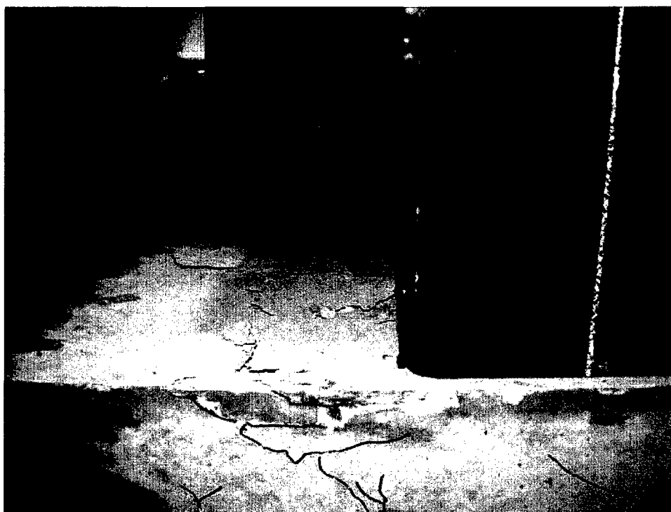
Figure 6. Concrete compression failure for Beam DS 18
