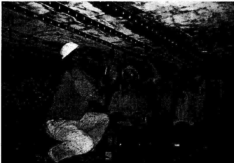
Figure 50. Fastening of the FRP strip at the midspan
