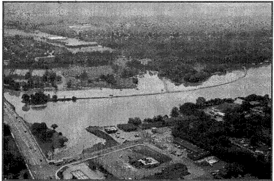
Figure 2. Aerial view of Drakes Creek restoration site (Phase 1)
