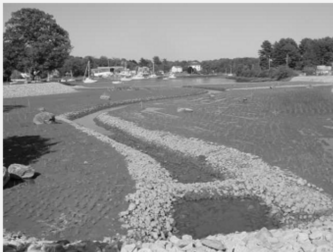
Figure 1 - Salt Marsh Establishment After Consolidation and Backfilling
