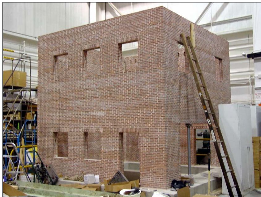
Figure 2-9. Completed test structure.
