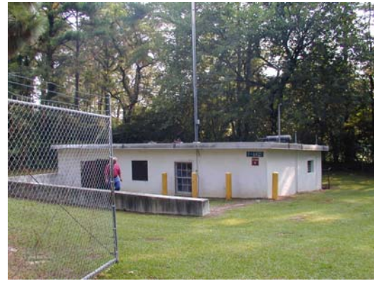
Figure 5. Fort Bragg upgrade—Lift Station #4.
