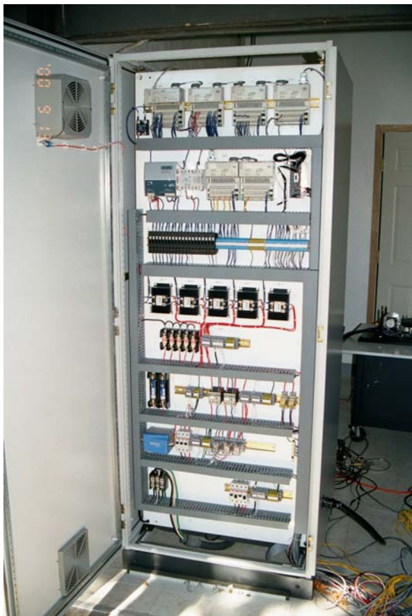
Figure 19. PLC control for the XCEM.
