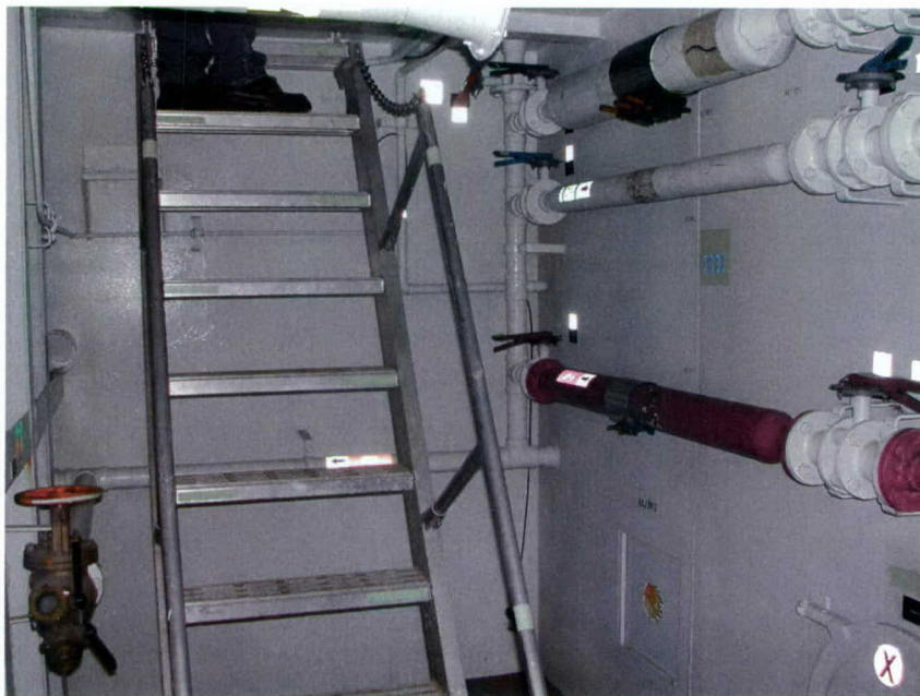
Fig. 2 – DCETF interior view of compartment A1 showing some of the “damages” and plumbing. The hatch to A2 is at the top of the ladder.
