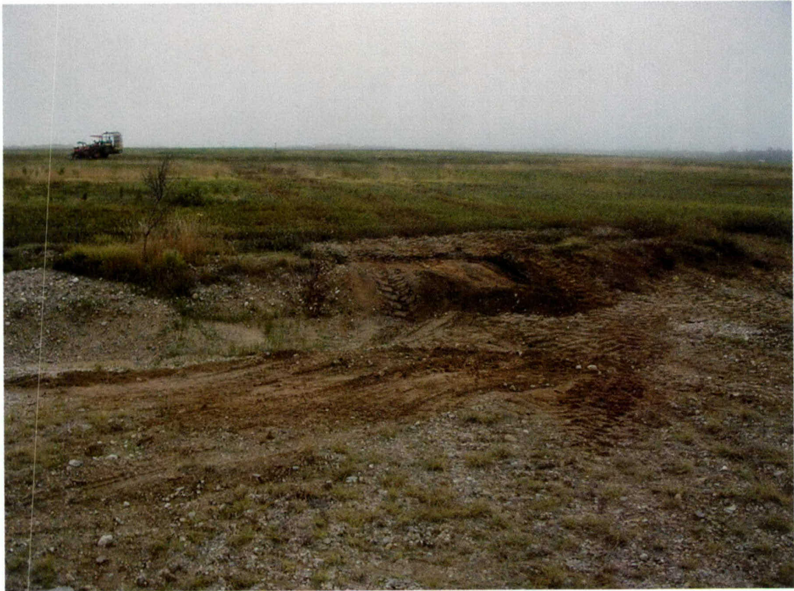
Plate 1. View east of soil erosion caused by blueberry harvesting equipment (in background) in Sector 1 at the Columbia Falls OTHB-E Radar Station.
