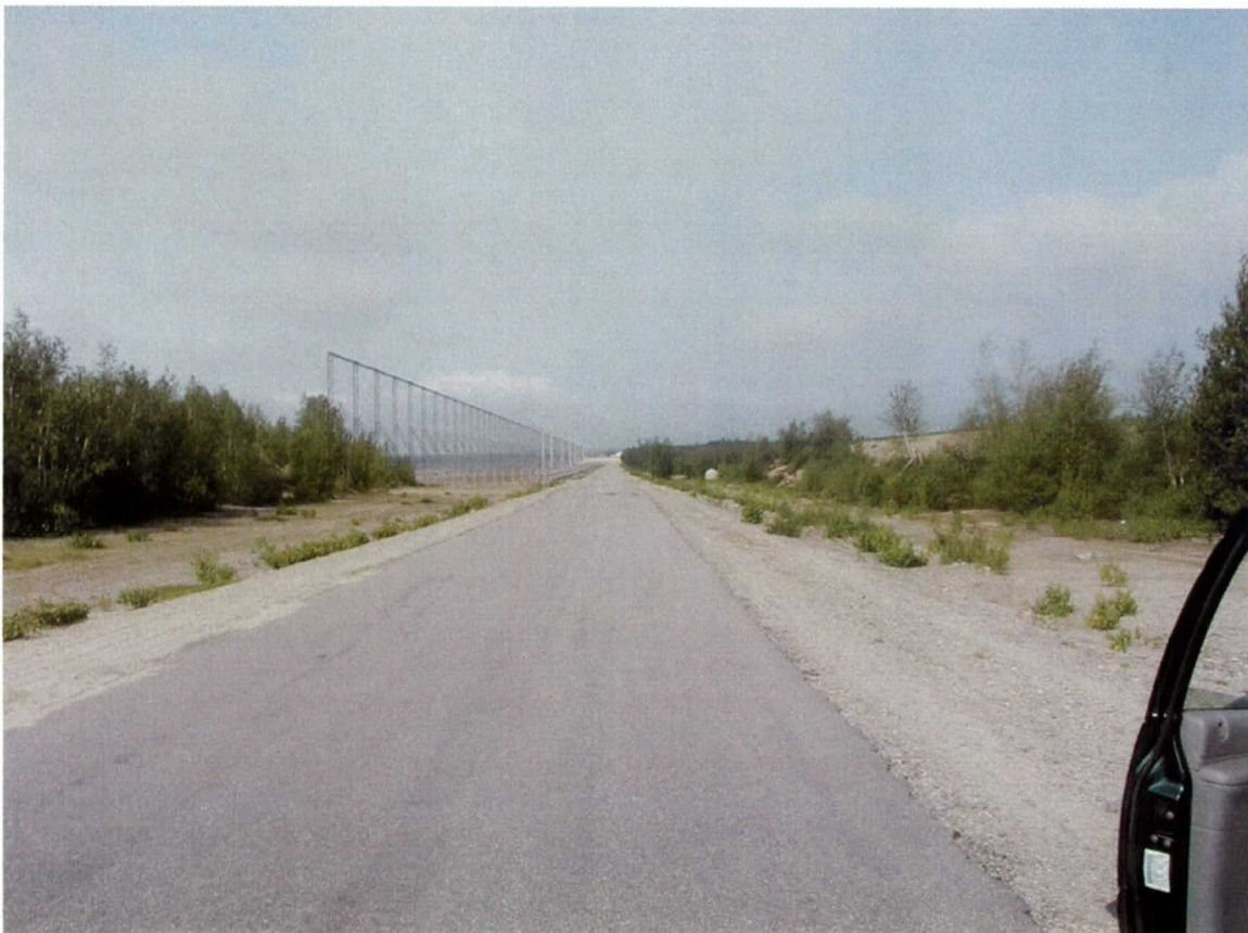
Plate 8. View west along northern perimeter road in Sector 3. The top of the cut bank (right) is property boundary and indicates the original ground surface elevation prior to construction.
