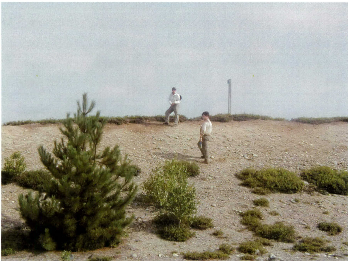
Plate 9. JMA crew conducting surface inspection of eroded cut bank in the eastern end of Sector 3. Note that the cut extended to the eastern property boundary (wooded post).
