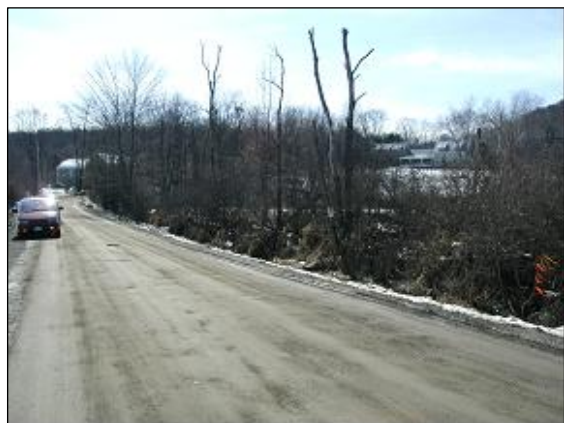
29 March 2002, Area 3, Geowrap, image 2.
