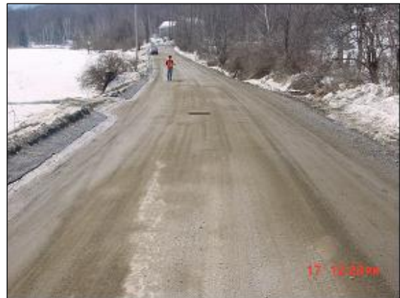
17 March 2003, Area 3, cement, image 2.
