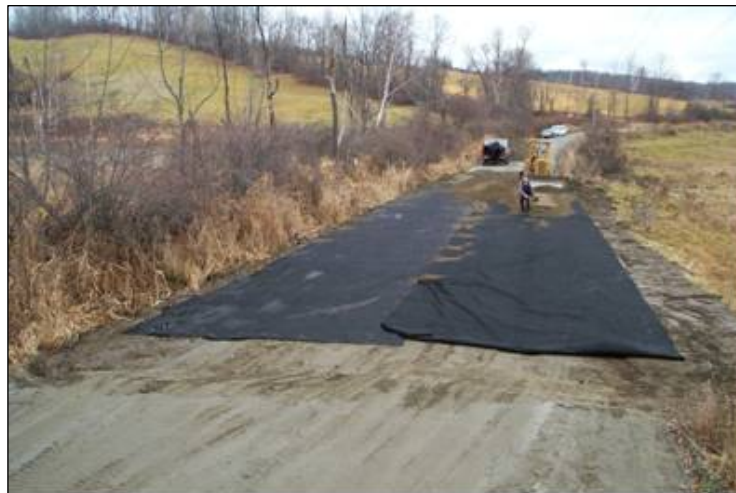
Figure 12. Top geotextile layer of geowrap during construction in Windsor, Area 3.
