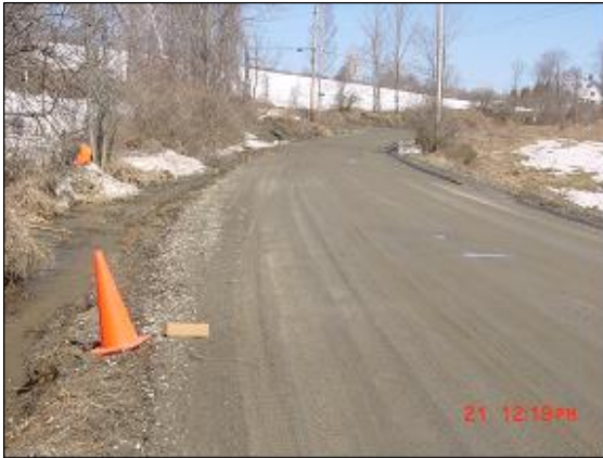
21 March 2003, Area 3, Cement, image 2.
