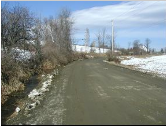
29 March 2002, Area 3, Cement, image 1.
