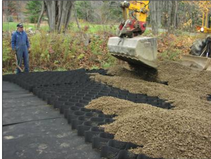
Figure 17. Geocell test section during construction.
