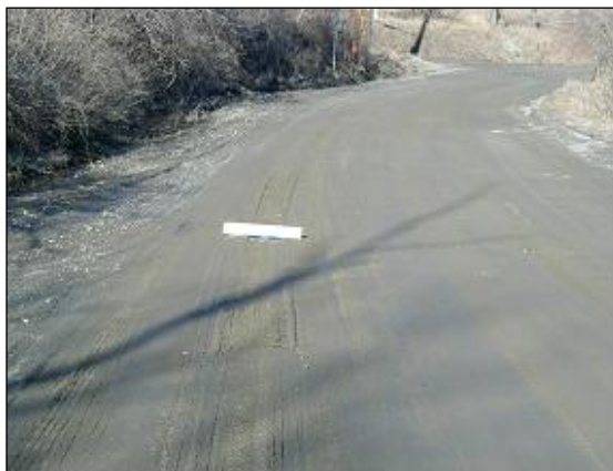
11 March 2002, Area 3, Cement, image 1.
