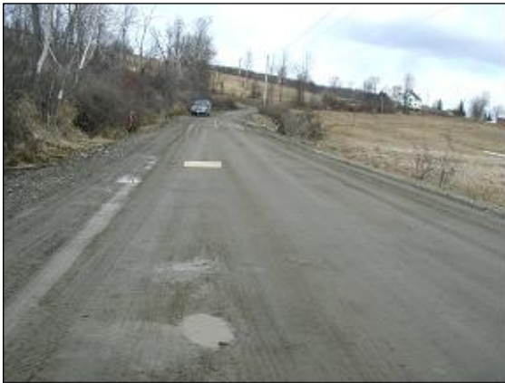
4 March 2002, Area 3, Geowrap, image 1.
