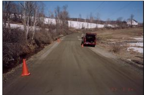
24 March 2003, Area 3, Geowrap, image 2.
