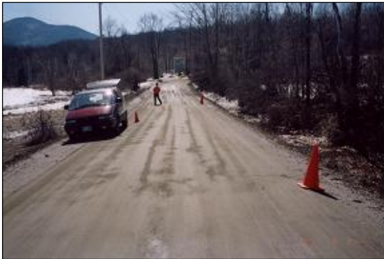
24 March 2003, Area 3, Geowrap, image 1.
