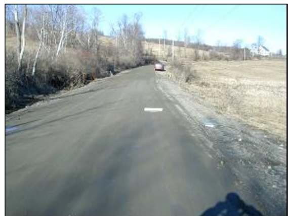
11 March 2002, Area 3, Geowrap, image 1.
