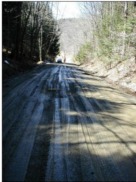
Figure 29. Control East (CE) of Area 4 on April 2, 2002, showing the differences in moisture content of the road surface due to degree of sun exposure.
