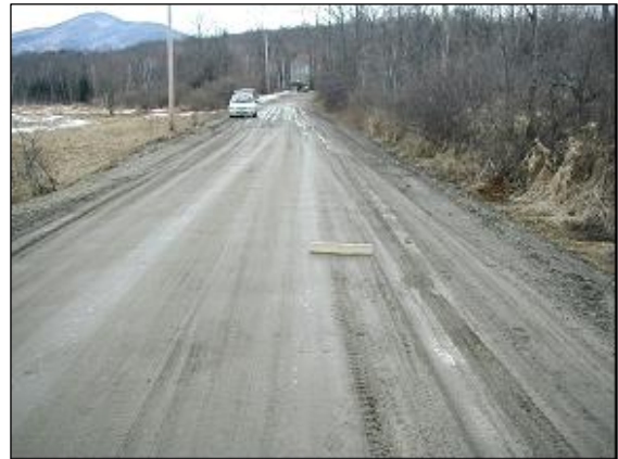
4 March 2002, Area 3, Geowrap, image 2.
