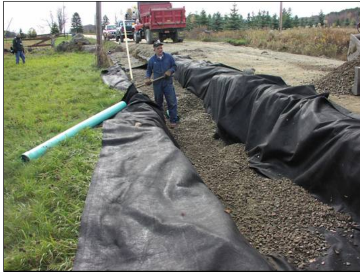
Figure 18. Westford Drain test section during construction.
