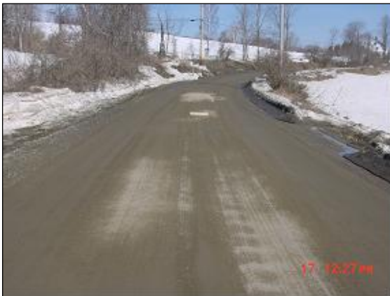
17 March 2003, Area 3, cement, image 1.
