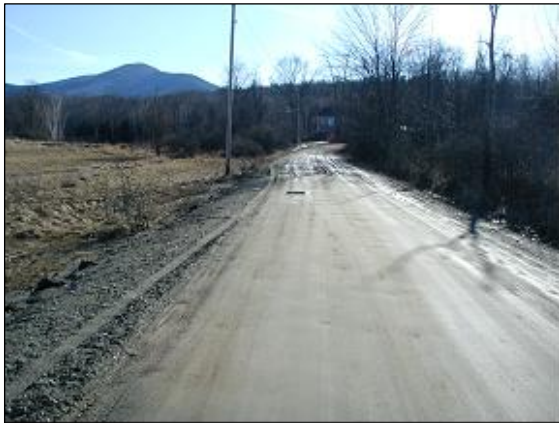
11 March 2002, Area 3, Geowrap, image 2.
