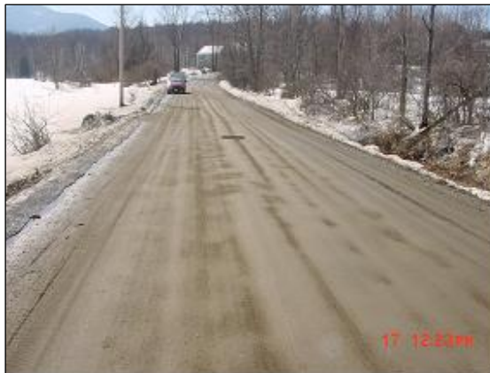
17 March 2003, Area 3, Geowrap, image 2.
