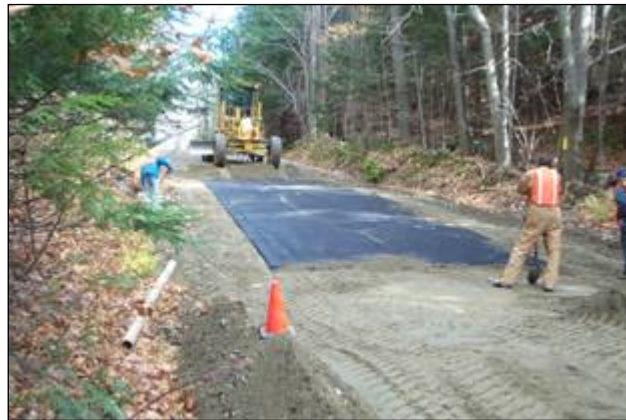
Figure 13. Geotextile separator during construction in Windsor, Area 4.
