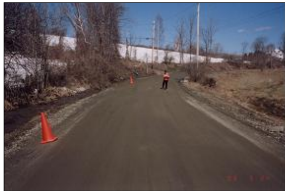
24 March 2003, Area 3, Cement, image 2.
