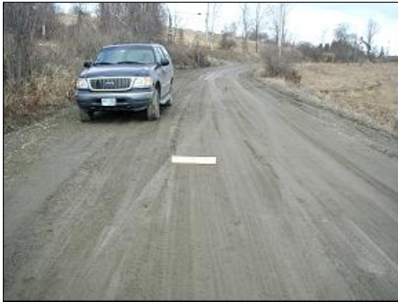
4 March 2002, Area 3, Cement, image 1.
