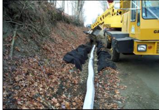
Figure 11. Installation of drainage in Windsor, Area 2. The image is looking west.
