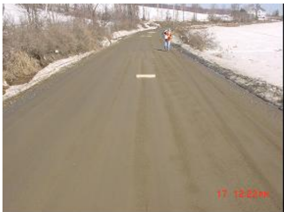
17 March 2003, Area 3, Geowrap, image 1.
