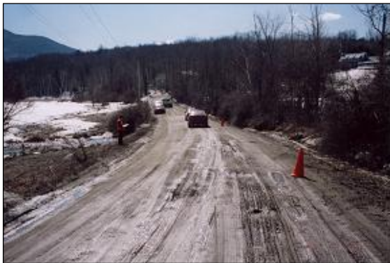
24 March 2003, Area 3, Cement, image 1.
