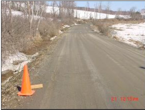
21 March 2003, Area 3, Geowrap, image 2.
