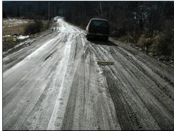
4 March 2002, Area 3, Cement, image 2.
