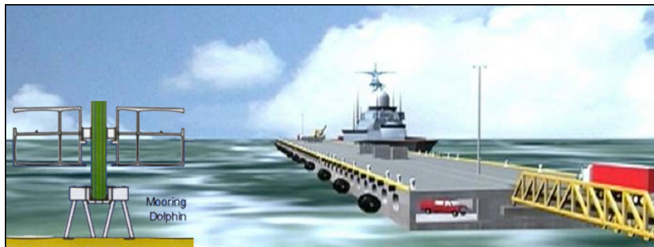
Figure 1 Modular Hybrid Pier
