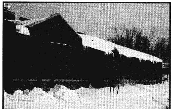
Figure 11: Both buildings from Figure 10 photographed at the same time. The unmodified building shown at the left was experiencing severe icings. The other building with improved attic ventilation had no icing problems.
