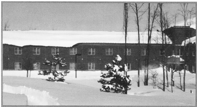
Figure 2: Some creep of snow and cornicing is evident, but no icings occurred on this roof.
