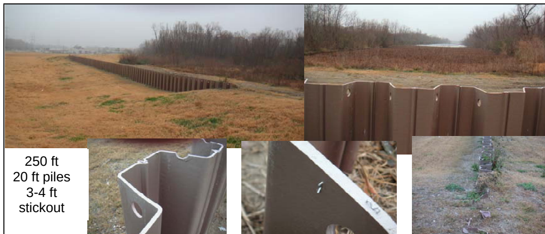
Figure 49. Vinyl sheet pile installed by the New Orleans District.
