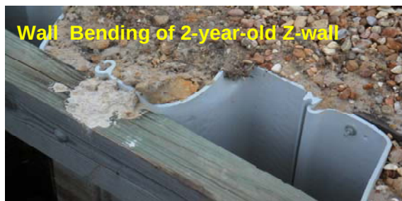
Figure 58. Examples of improper structural designing of PVC sheet pile showing buckling of the pile web, bending of the wall, and interlock failure.
