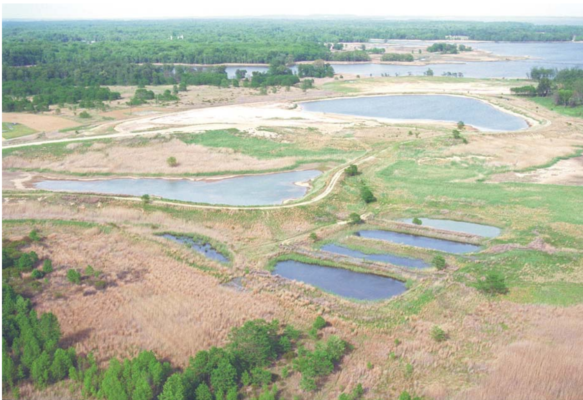
Figure 12 – Oblique aerial photo of part of the dewatering ponds. The four small ponds in the foreground and the larger pond above were included in this survey.
