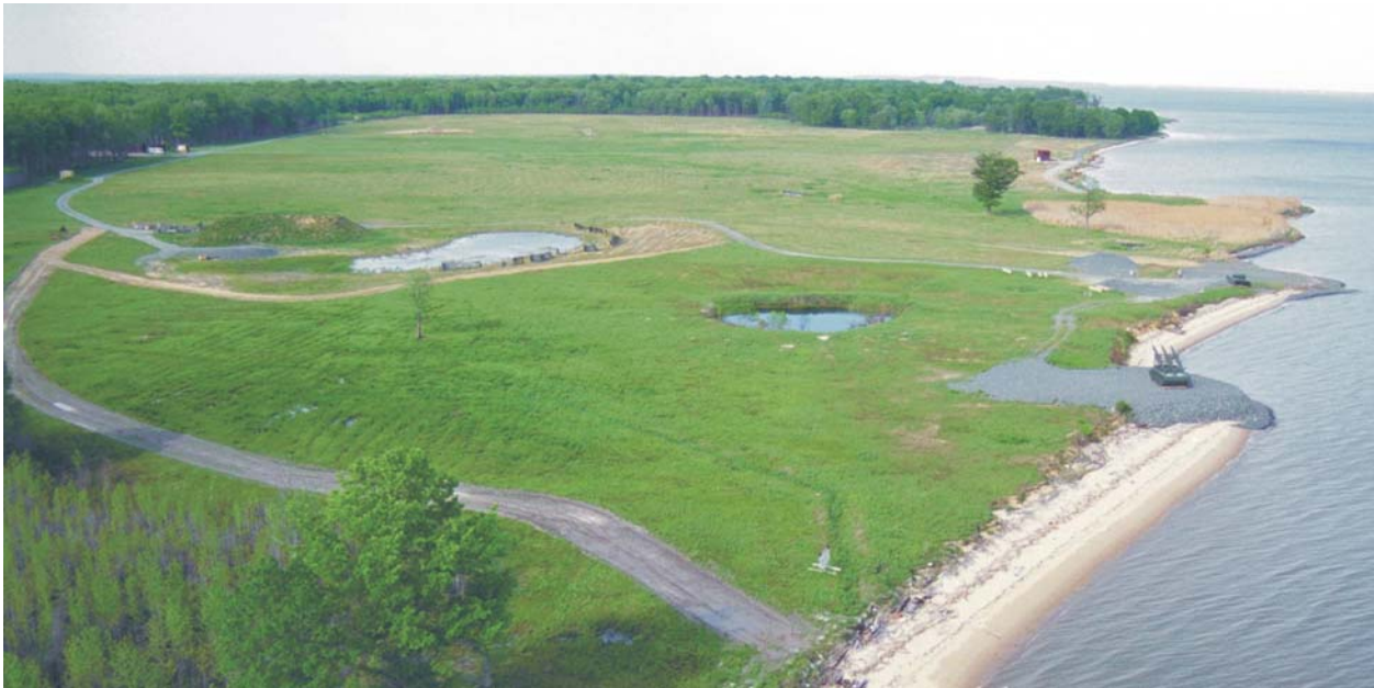
Figure 16 – Aerial photo, looking approximately west to east, shows the Active Recovery Field. The Impact Area includes the cleared area and offshore areas that may extend for an additional several hundred meters.
