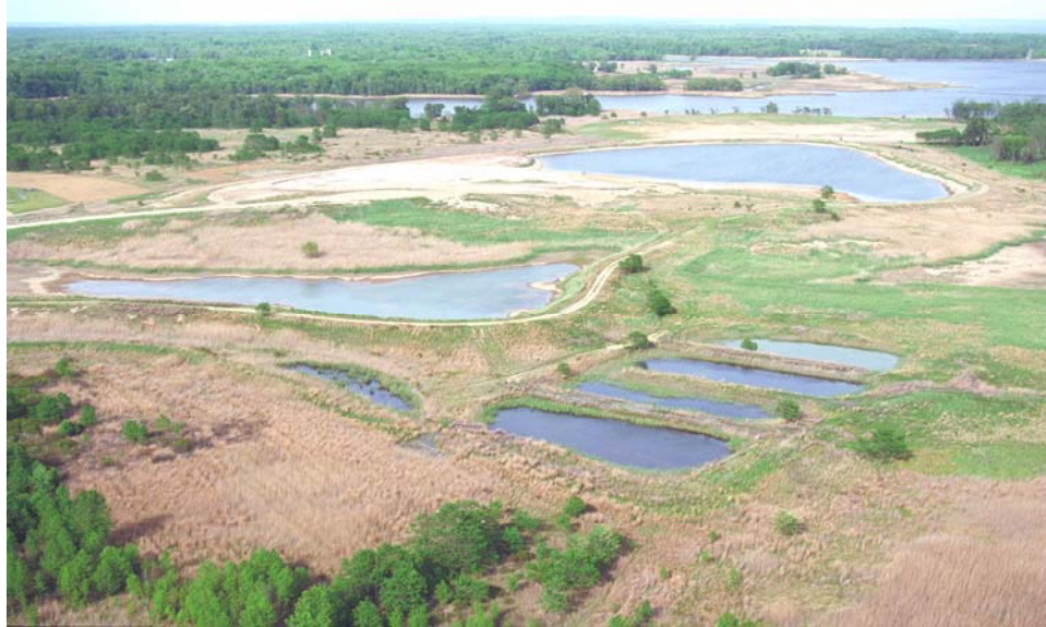
Figure 19. Dewatering Ponds Area [2]
