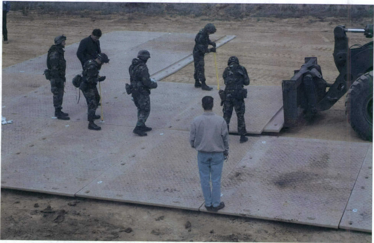
Photo 10. Dual-use bar tool used to align panels and lock in connector pins
