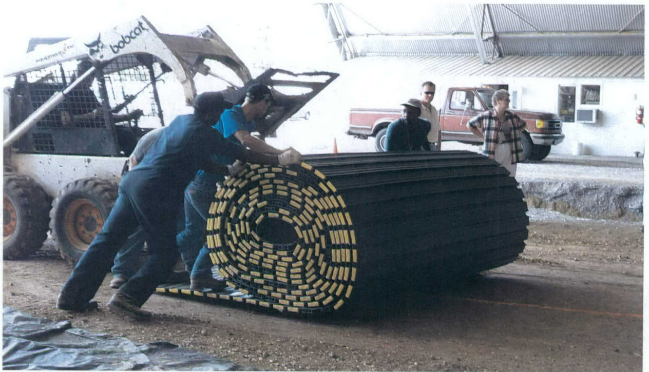
Photo 29. Installing Rolla-Road matting system
