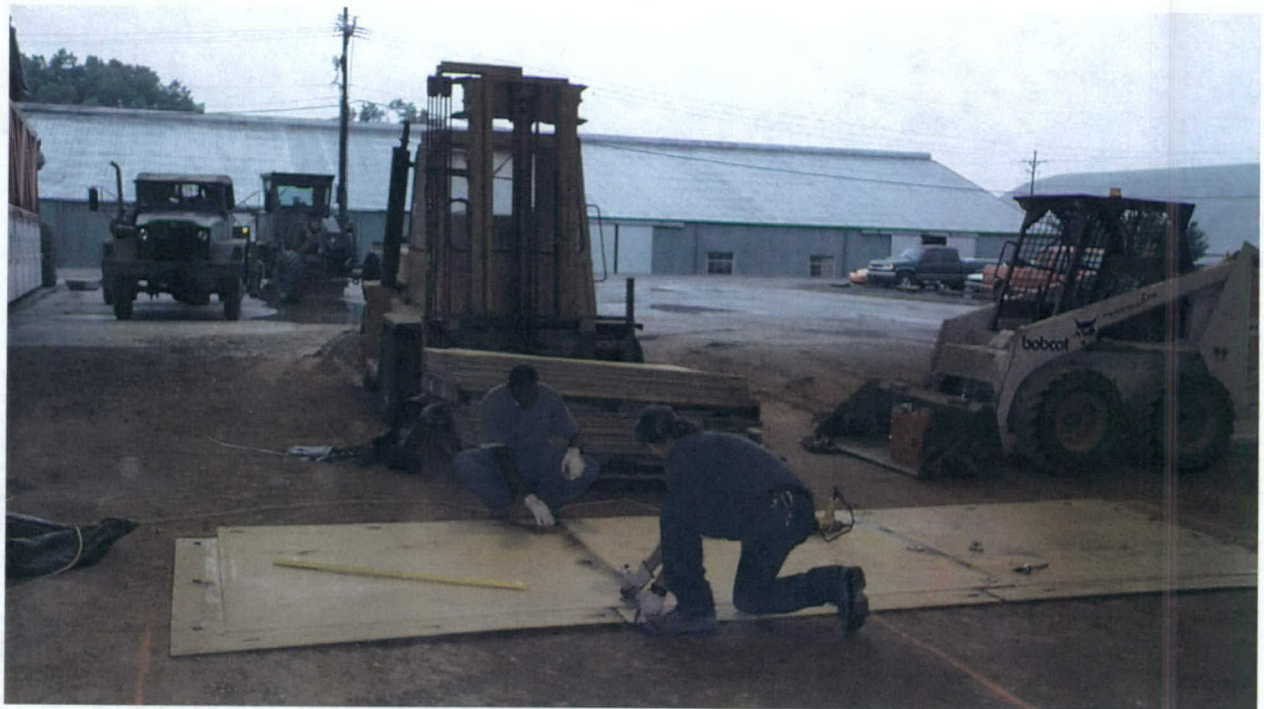
Photo 27. Installing 5-ply MP matting system
