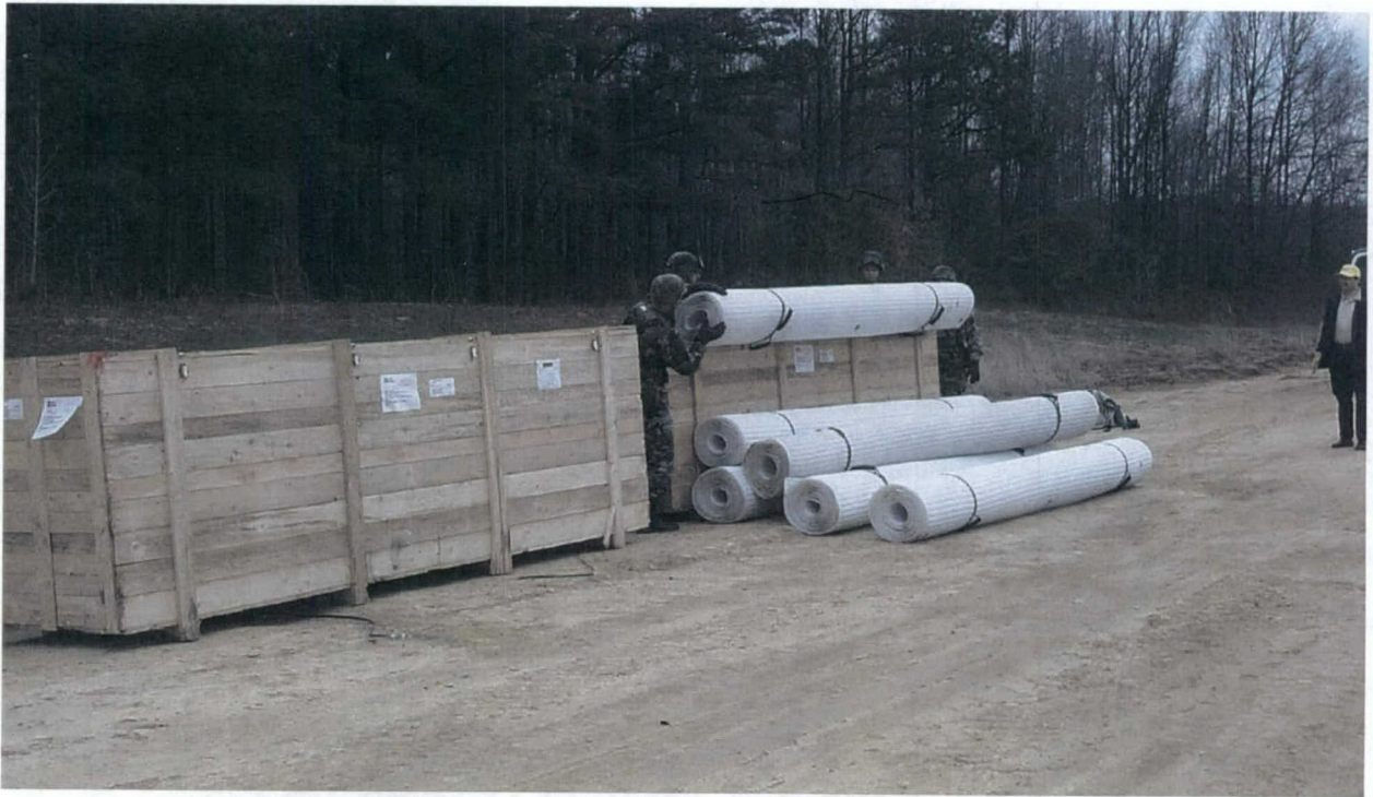
Photo 3. Unloading rolls of Mobi-Mat from shipping crates
