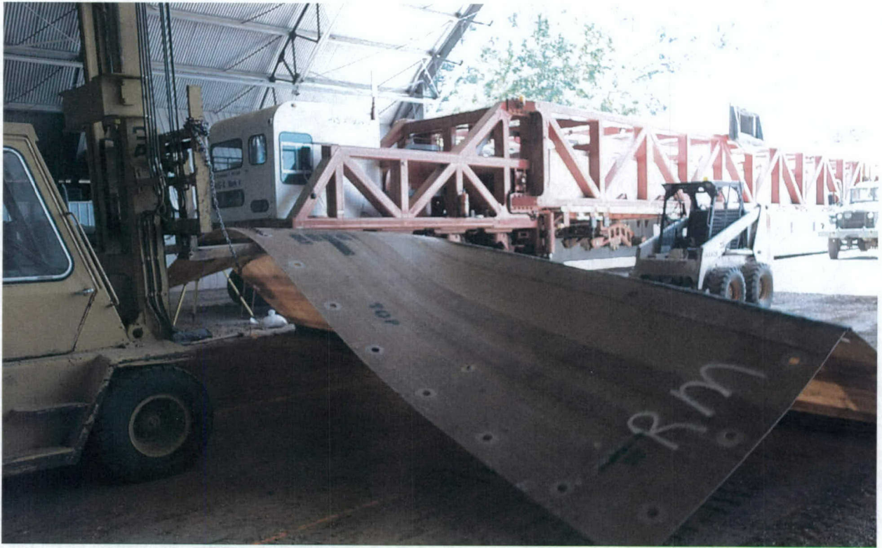
Photo 28. Installing Rapid Mat (FPM) matting system
