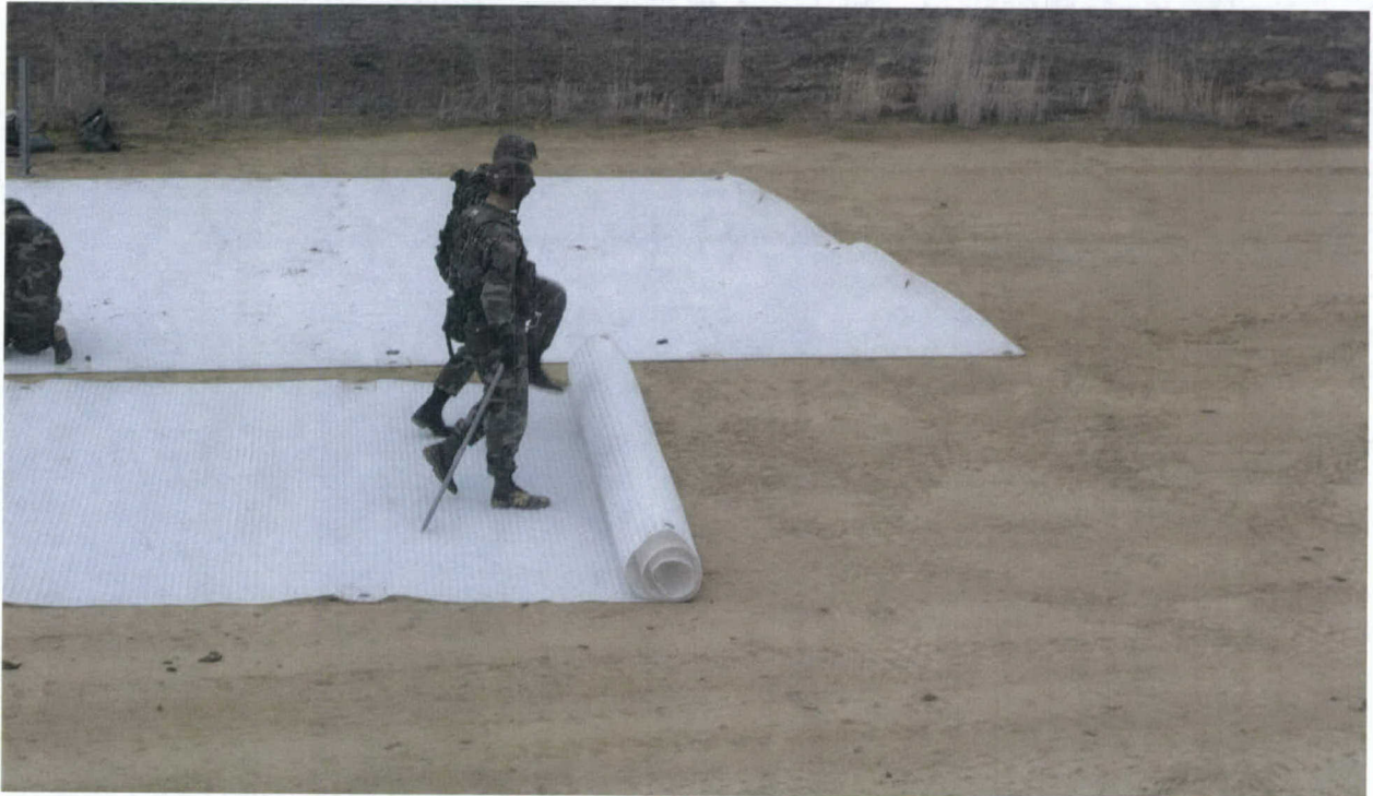
Photo 4. Rolling out Mobi-Mat before anchoring to adjacent panel and staking edges
