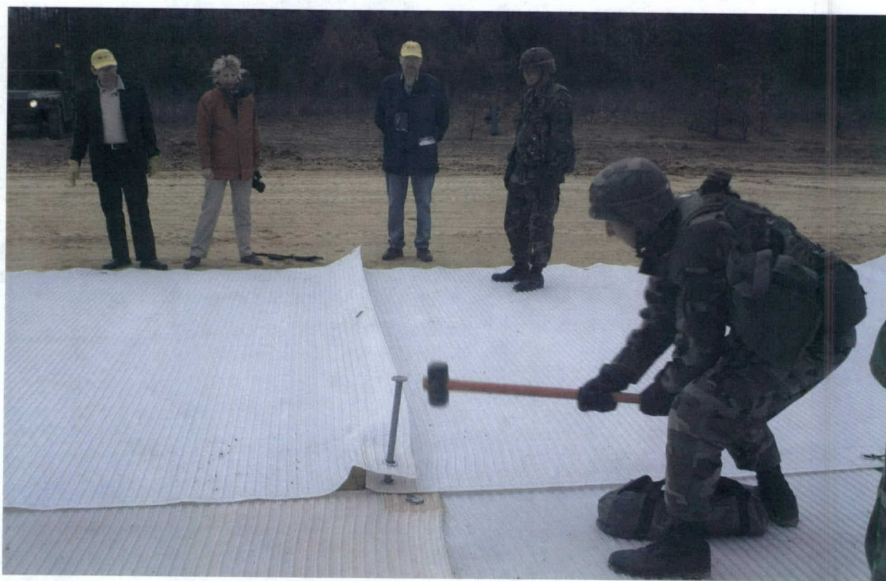
Photo 6. Hammering corner stakes into Mobi-Mat panels
