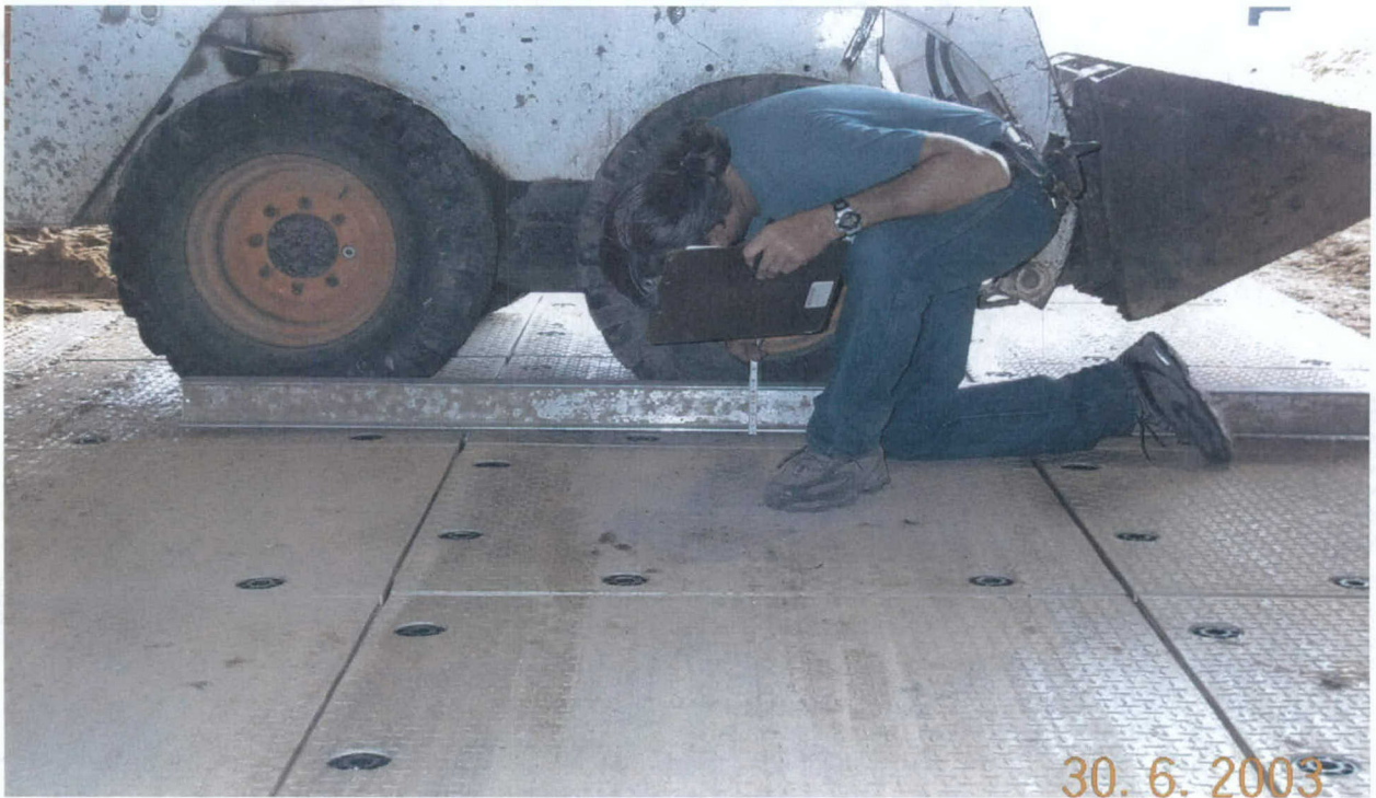
Photo 36. Using the skid-steer multipurpose machine to measure mat in-place rutting
