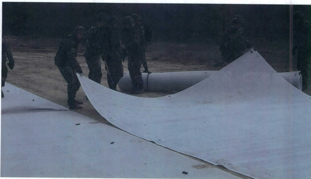
Photo 5. Stretching out Mobi-Mat panel before anchoring
