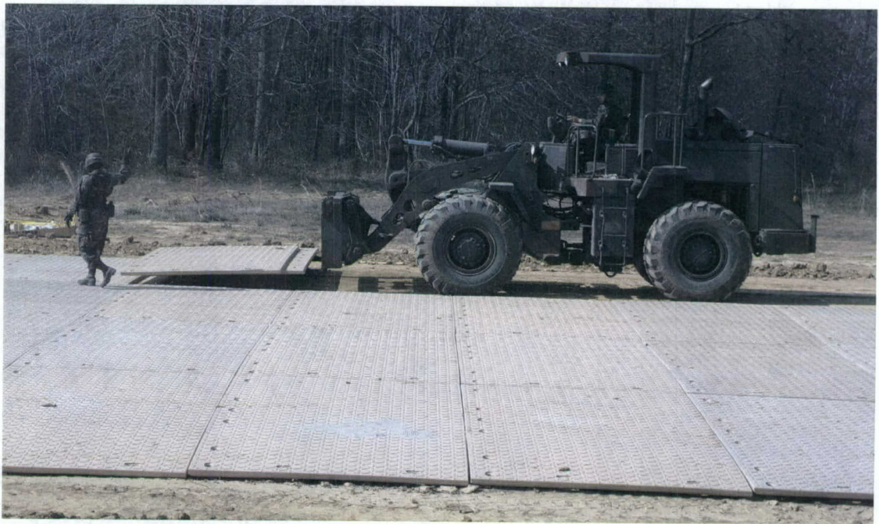
Photo 8. Large forklift used to place each DURA-BASE panel
