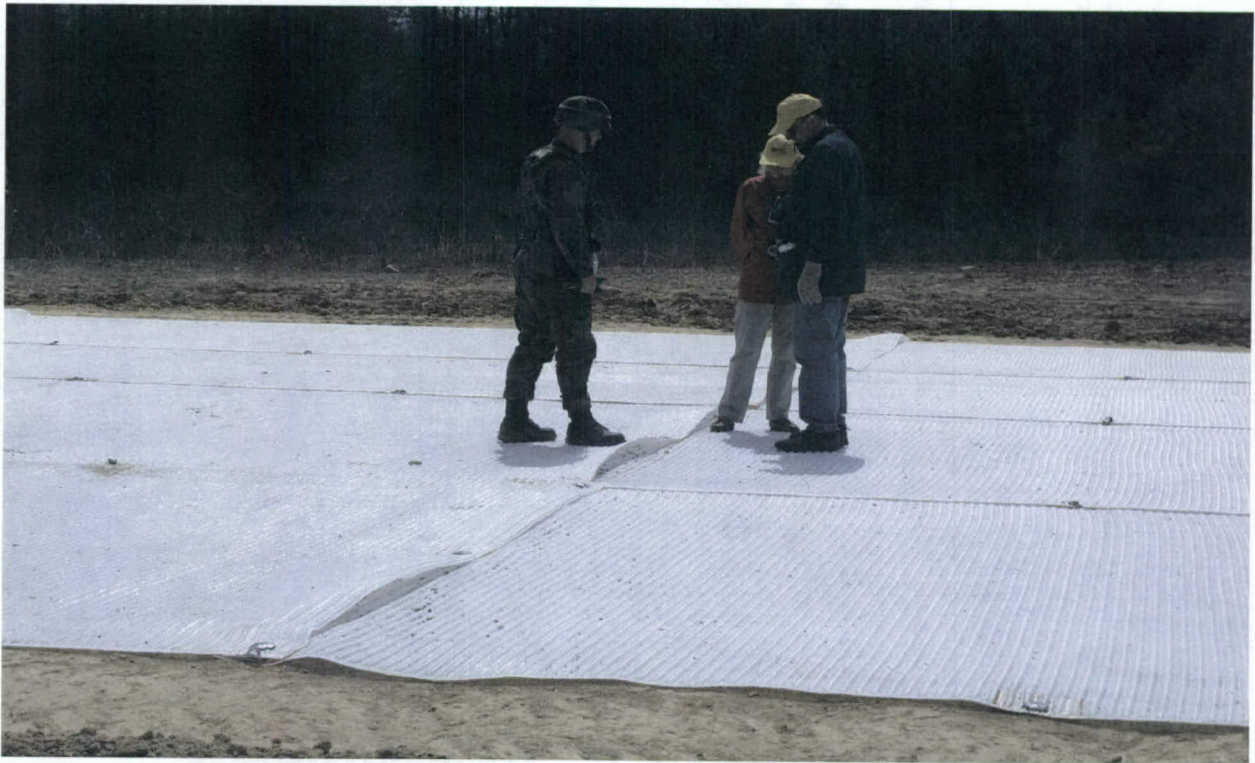
Photo 7. Completed Mobi-Mat helipad. (Note tops of pins used to hold it in place)
