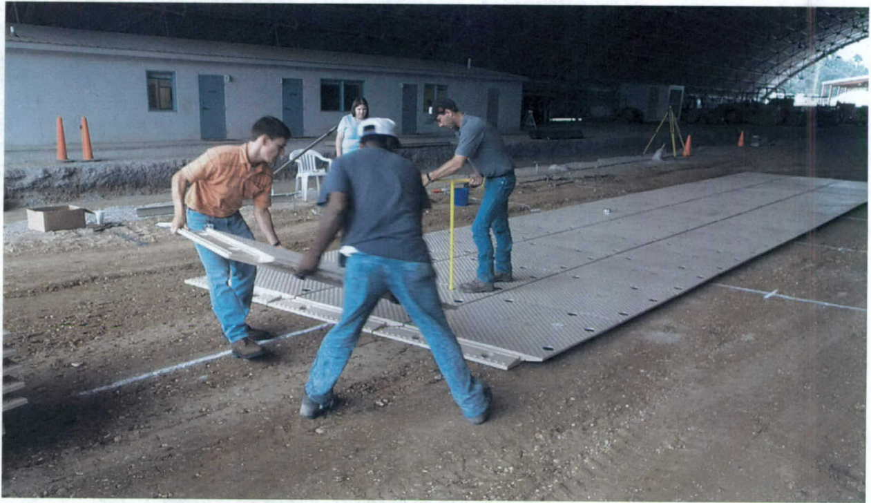
Photo 30. Installing SP-12 matting system
