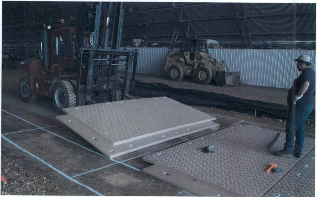
Photo 26. Installing DURA-BASE matting system
