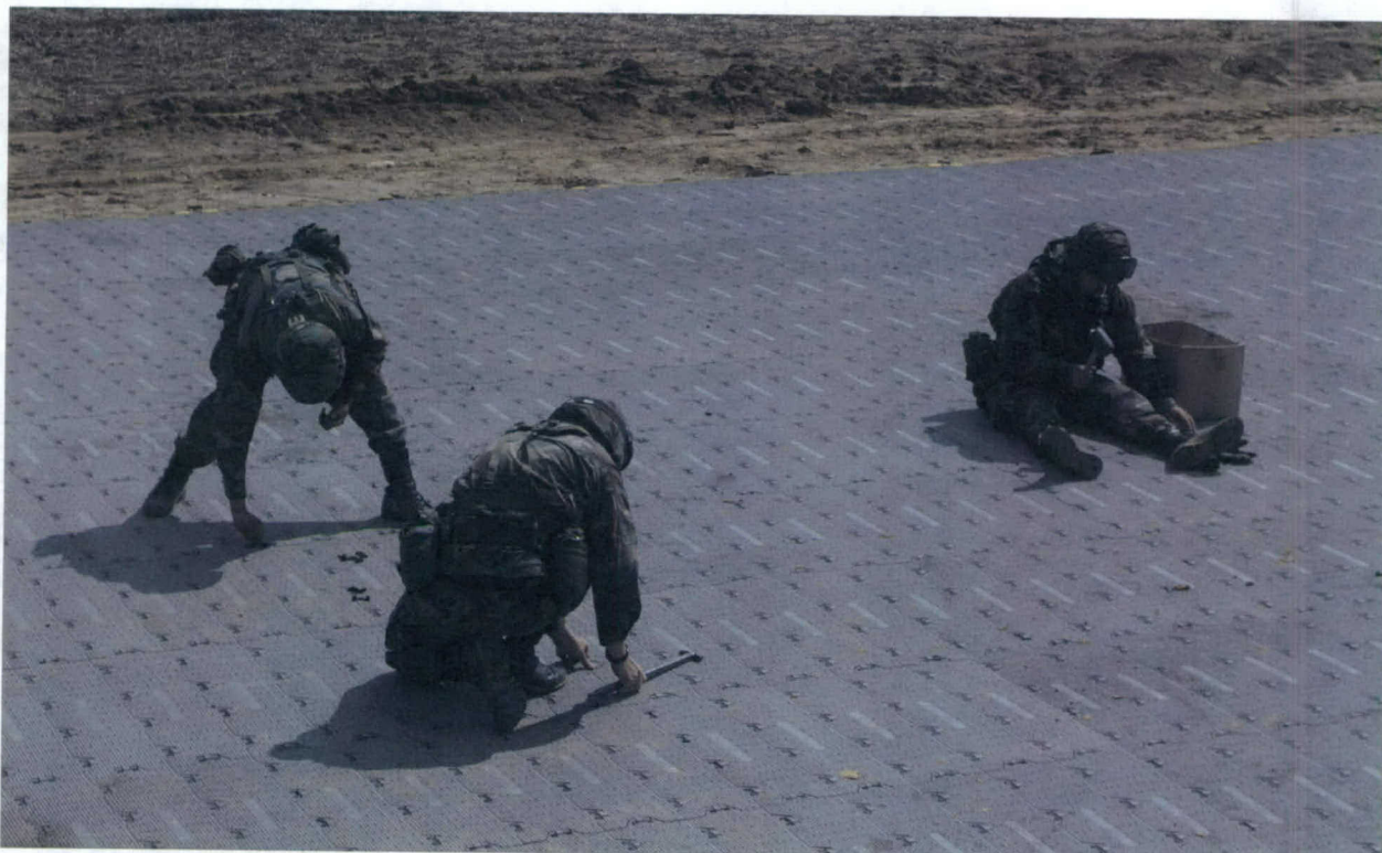
Photo 13. Tapping in SUPA-TRAC connector pins
