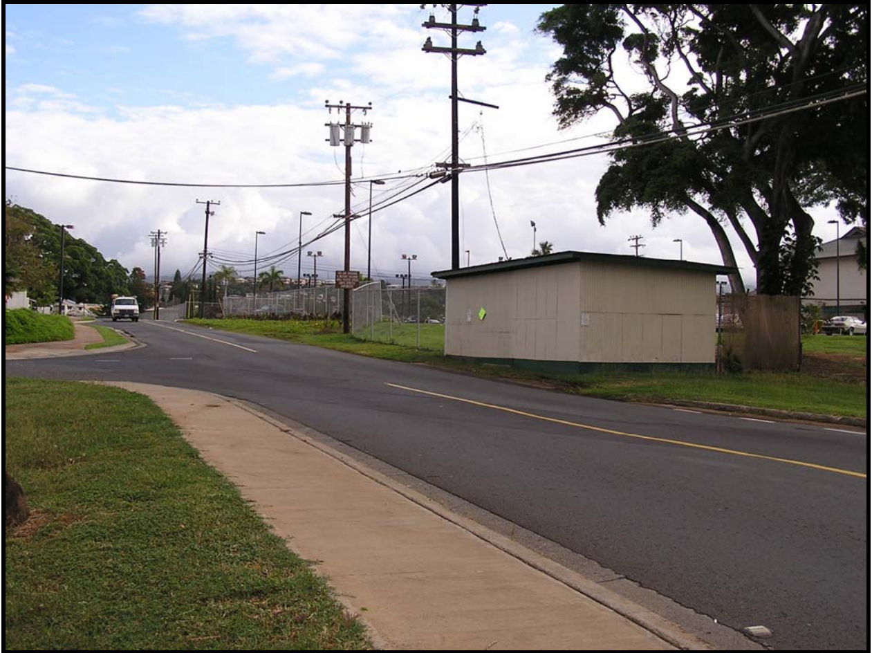
Figure 3-3 Pump House Located East of Warden Ave. at Valkenburgh St. Intersection
