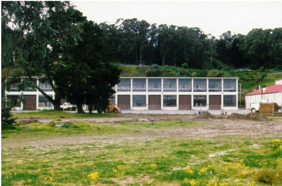
Figure 3. Site disturbance resulting from poorly planned staging of construction materials (source, R. Young).
