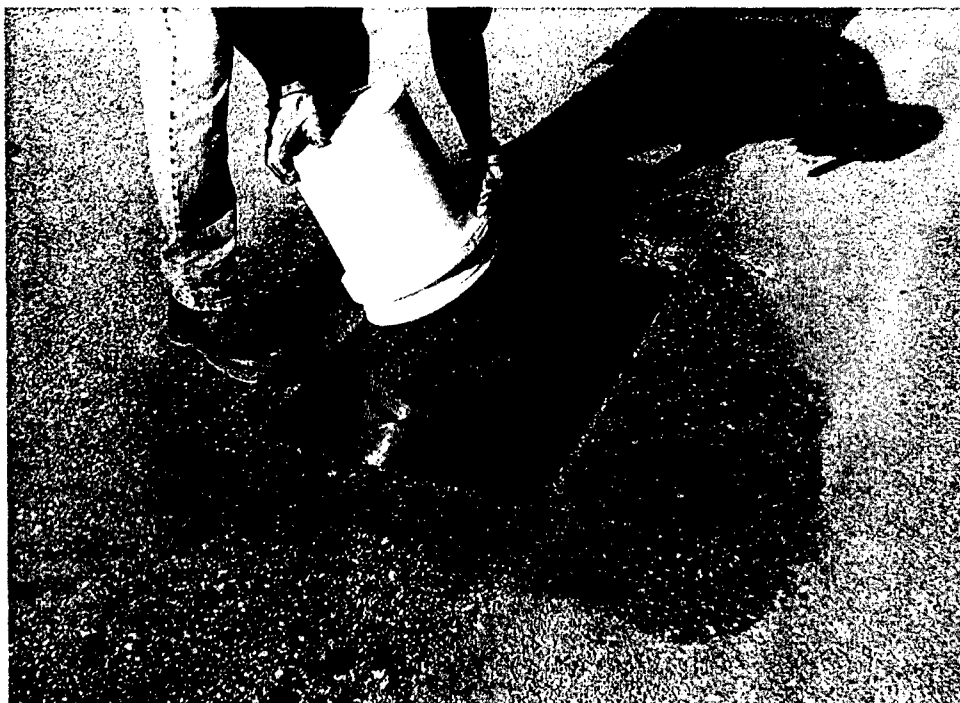
Figure 17. Adding cold-mix patch material to a hole filled with water
