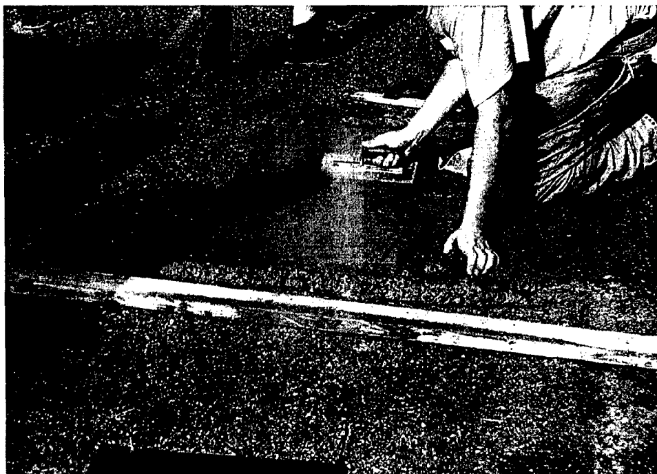
Figure 12. Finishing a patch with a trowel
