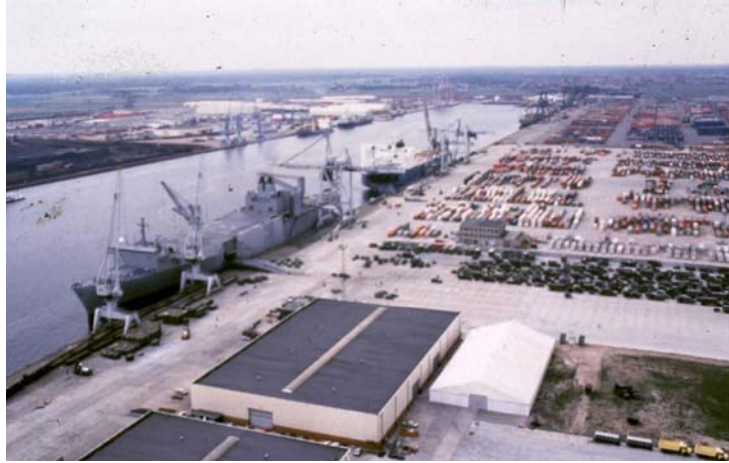
Figure 1. Seaport of Embarkation (SPOE). Cargo in the marshalling yard is positioned for loading on to ships. Each ship has storage areas, or compartments, that are each dedicated to one type of cargo load, including some subset of breakbulk; container; lift-on, lift-off (LOLO); roll-on, roll-off (RORO); and petroleum, oil and lubricants (POL). Some ships have their own cranes, while others depend on port material handling equipment. Compartment capacities for breakbulk and container loads are expressed in measured tons, while LOLO and RORO are in square feet.
