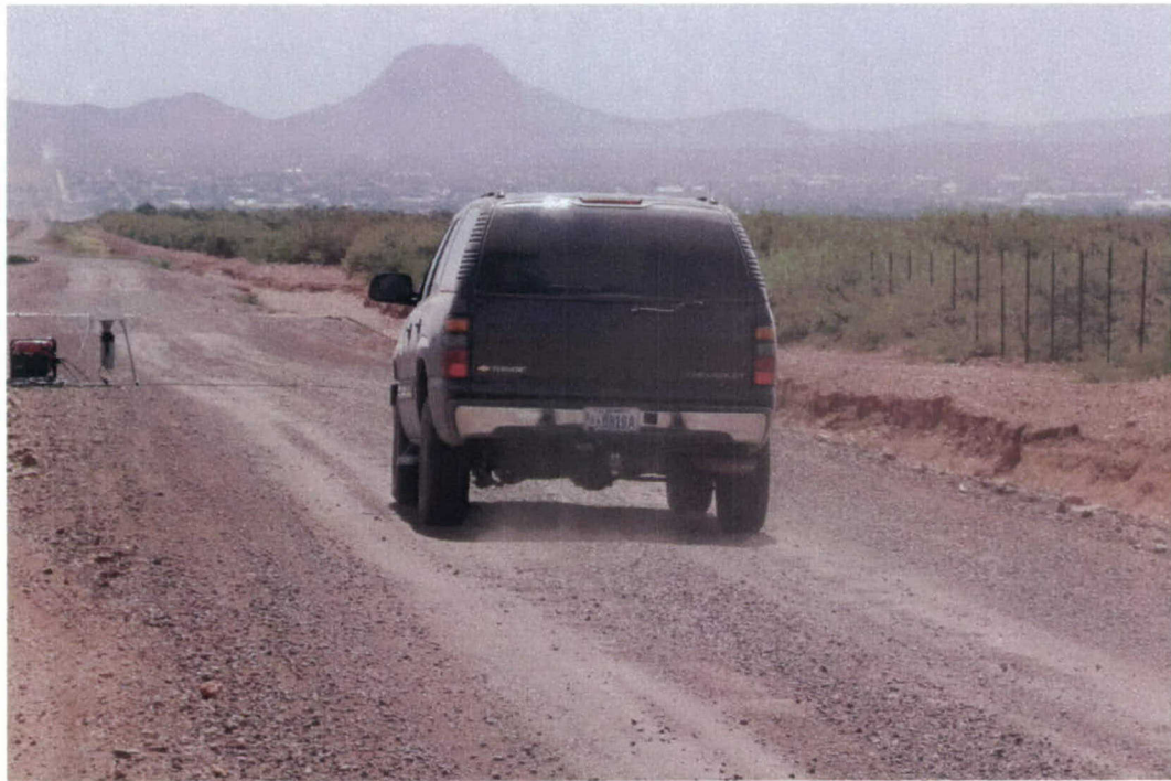
Photo 46. Good dust abatement on Section 19, Soiltac®
