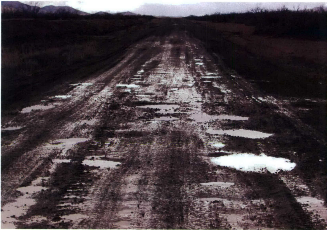
Photo 1. Initial road surface condition
