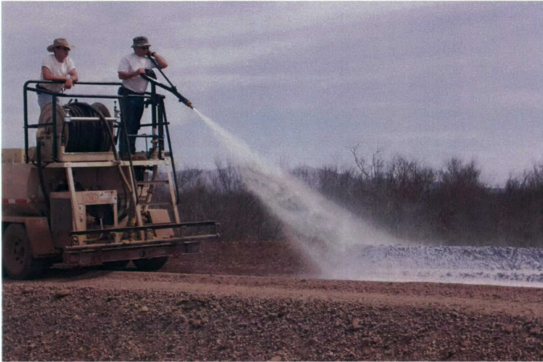
Photo 13. Spraying product on windrows using hand wand
