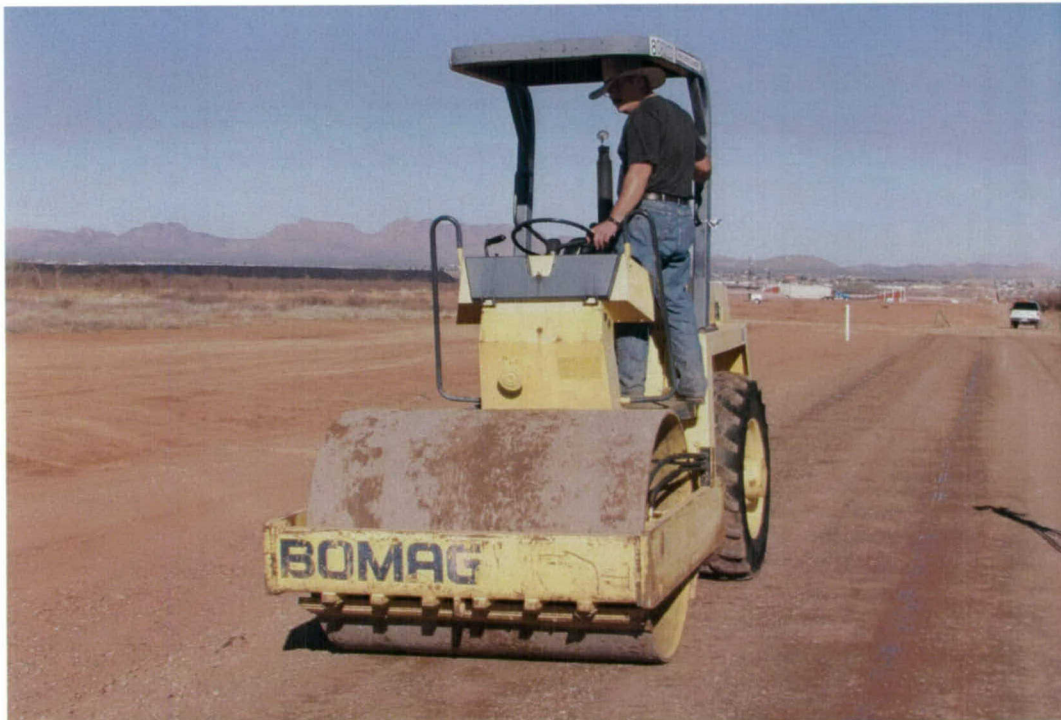
Photo 8. BOMAG 6-ton steel wheeled vibratory compactor
