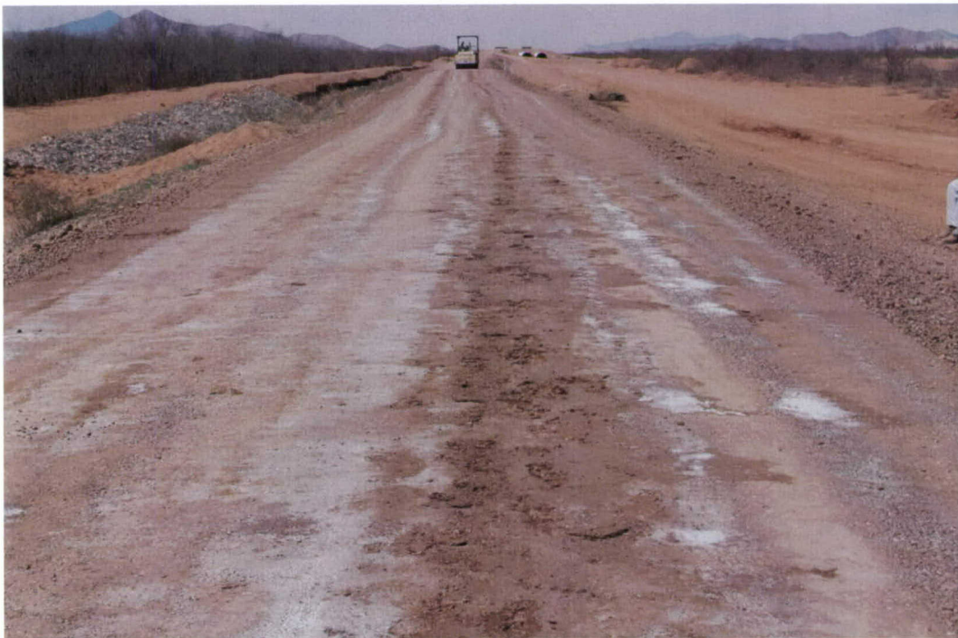
Photo 16. Rough surface on Section 3 caused by removal of tacky surface during compaction
