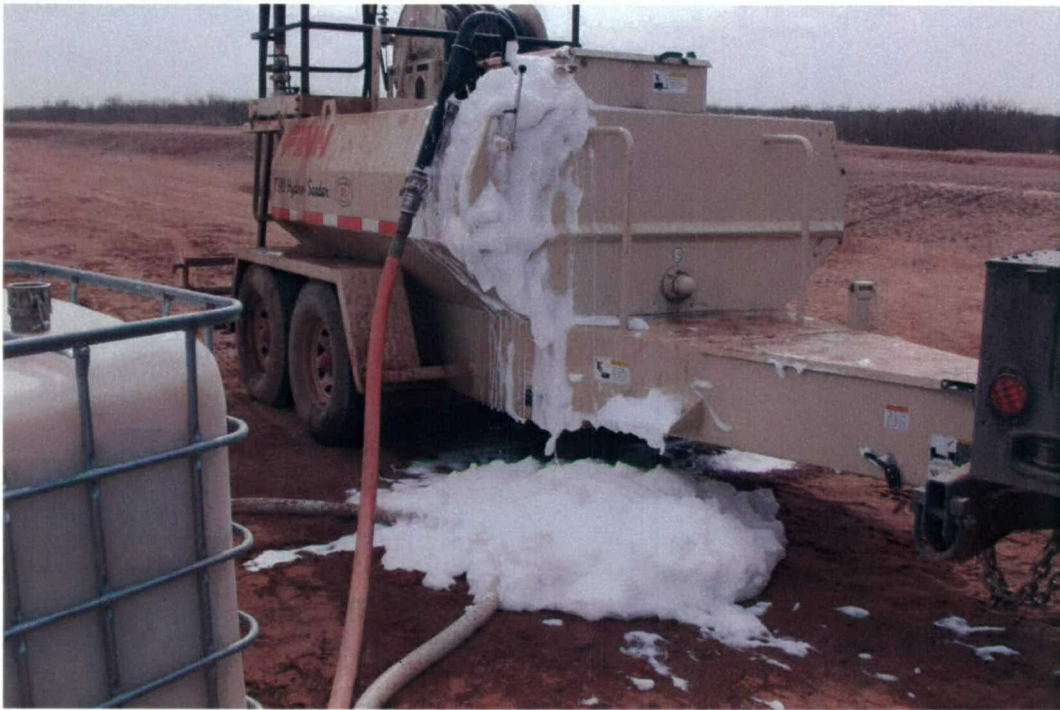
Photo 33. Foam overflowing hydroseeder while filling with Polytac®
