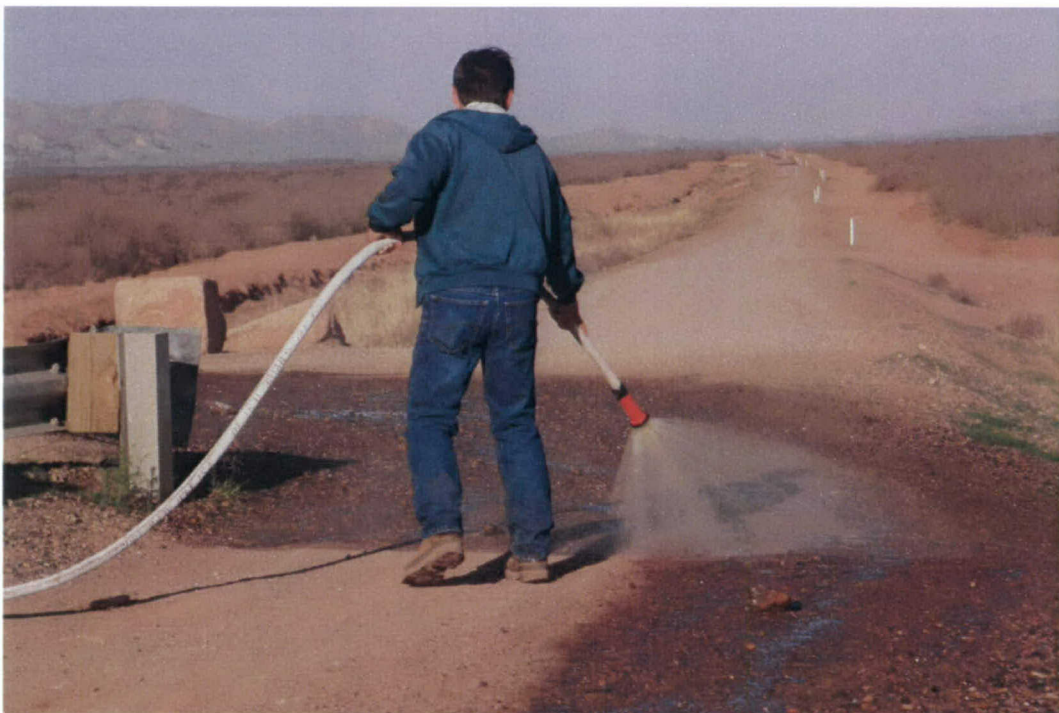
Photo 30. Applying EK-35® with hand wand on E-Spray system
