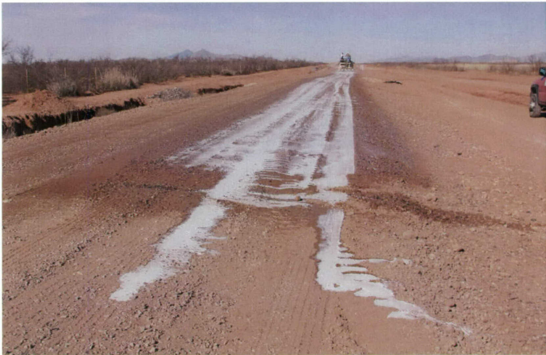
Photo 12. Delayed penetration and product runoff on section 2
