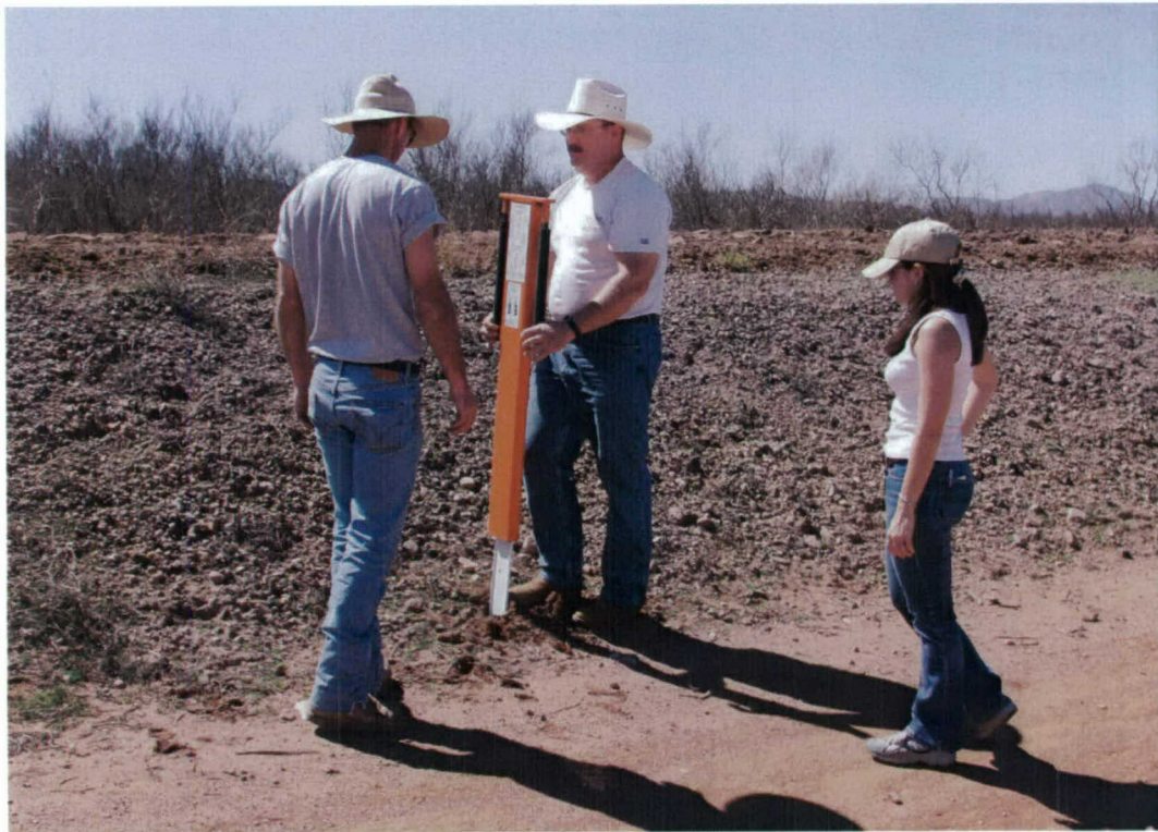
Photo 4. Placement of traffic delineators
