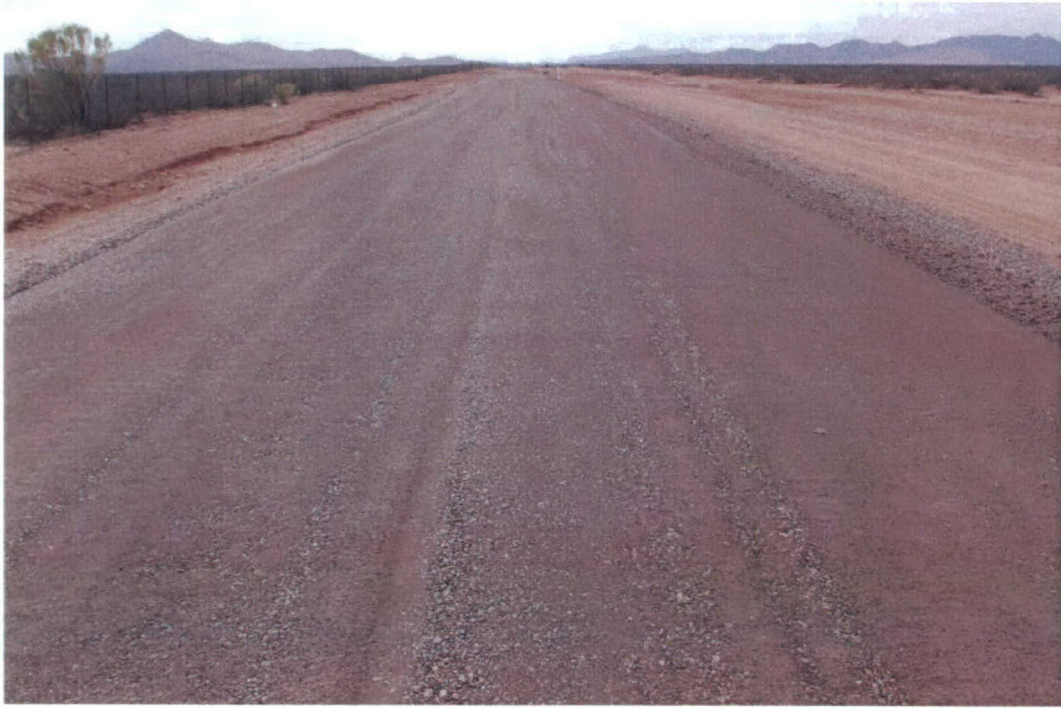
Photo 21. Final road surface after topical application
