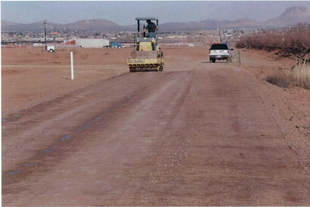
Photo 11. Section 1 after compaction
