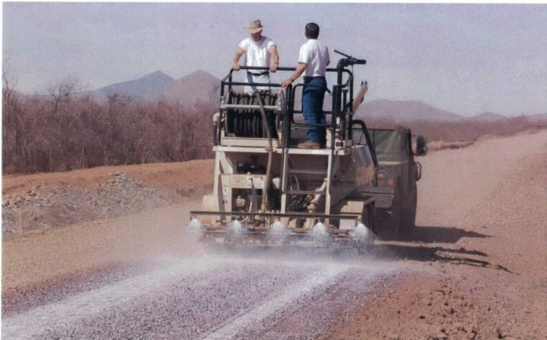
Photo 10. Spraying from distribution bar on hydroseeder
