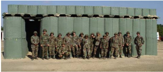
Figure 1. Hesco Bastion personnel bunker
