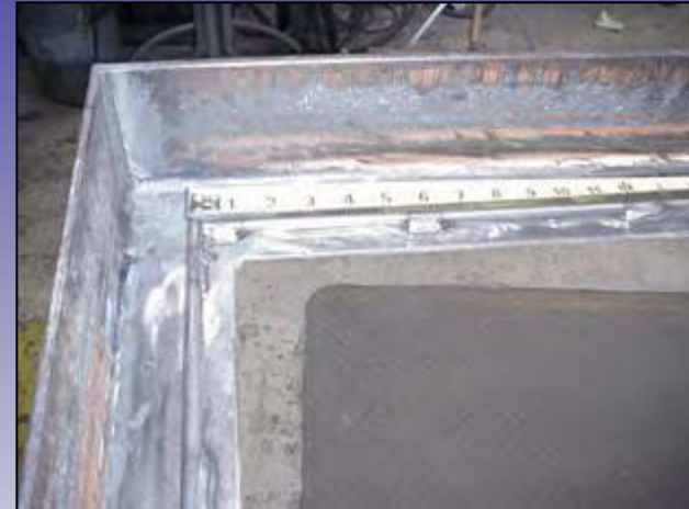
Rods Welded on Frame
