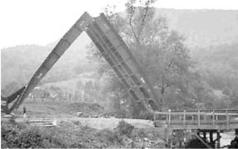
Army engineers reinforce a damaged timber trestle bridge with an armored vehicle launched bridge and . . .
