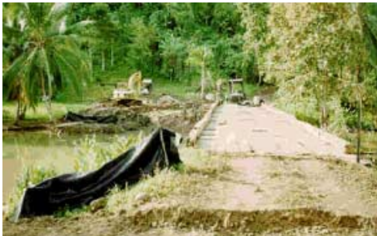
Marine engineers performing road and bridge construction.
