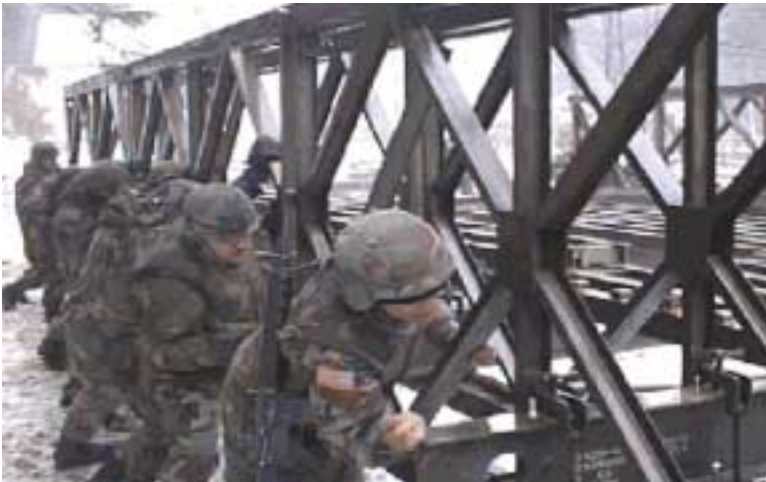
. . . Navy SEABEES assemble a Bailey bridge in Bosnia.
