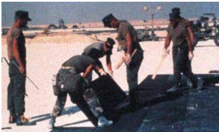
Navy SEABEES place airfield matting for helicopter apron during Operation DESERT STORM.
