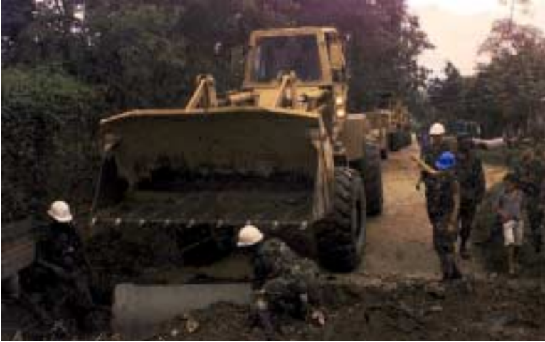
Army engineers install culvert in El Salvador.
