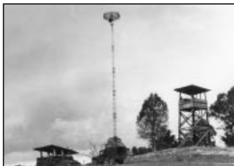
■ Camp Sentinel Radar.
