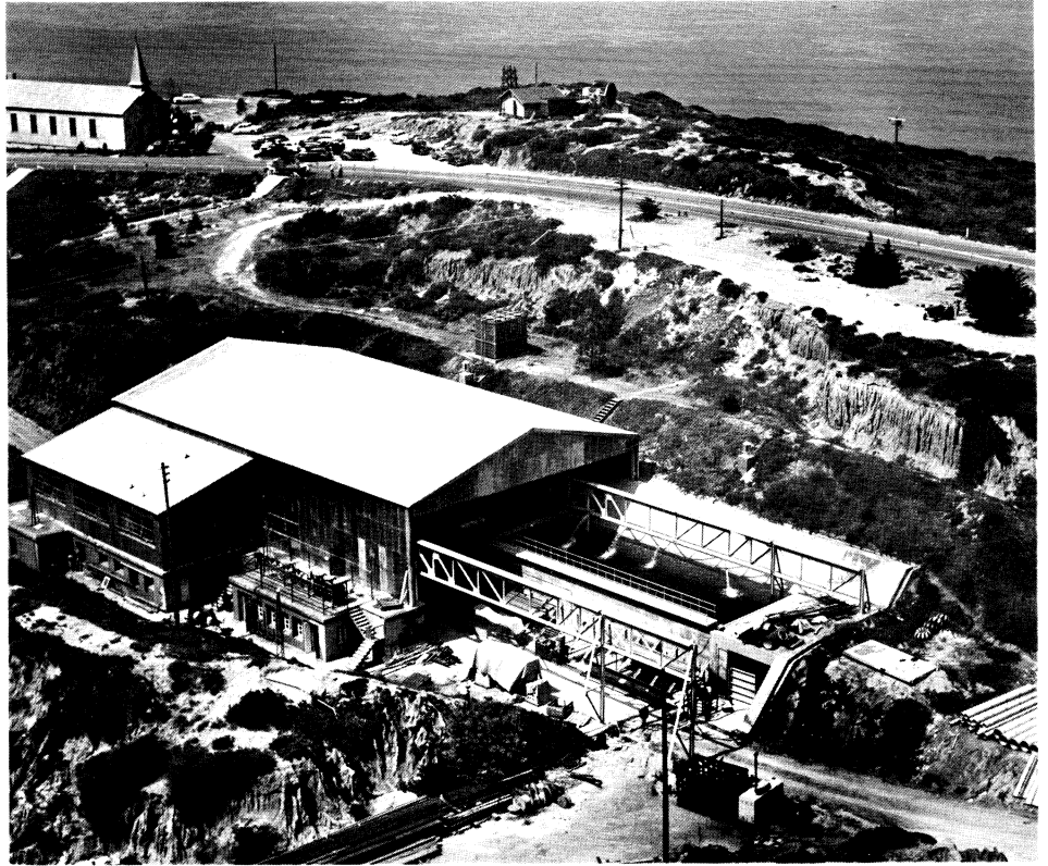
Battery Whistler after conversion for use by NEL. The old mortar battery was converted to a laboratory for testing the effects of seawater and different water pressures on materials devices used by submarines.
