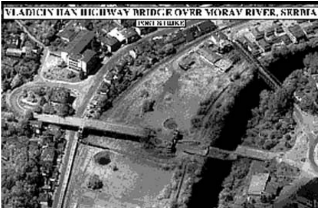
Destroyed highway bridge over the Morav River, Serbia
