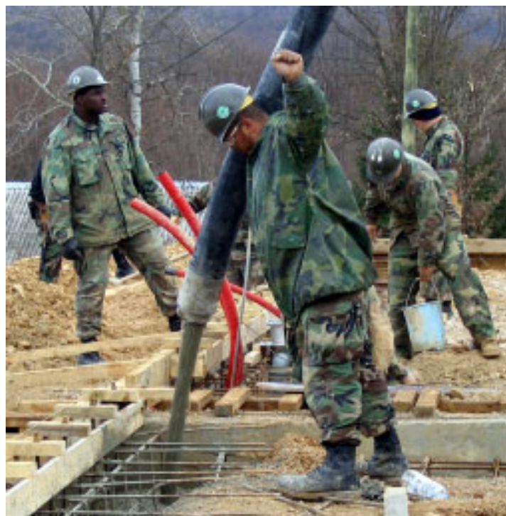
Humanitarian and civic assistance as part of a foreign internal defense program includes engineering construction projects.
