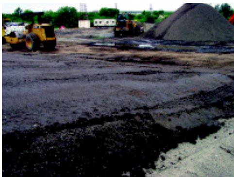
Compacting the blended mixture
