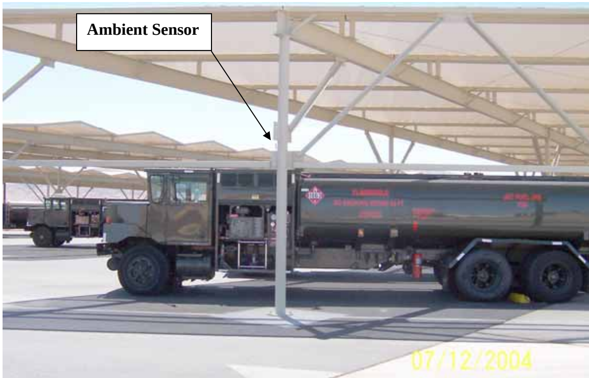
Figure14: Location of ambient temperature data logger.
