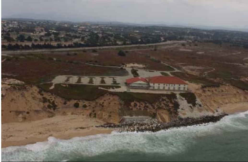
Figure 7. Oblique aerial photograph of Stillwell hall in 2002 in Marina, CA. The rock revetment can be seen at the base of the dune and marked erosion can be seen on either side of the revetment. Photograph copyright © 2002 Kenneth & Gabrielle Adelman ( http://www.californiacoastline.org/ ).
