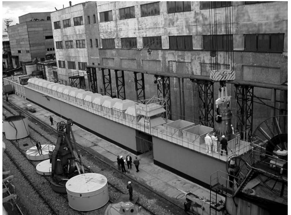
Figure 4: Interim Storage Pad
