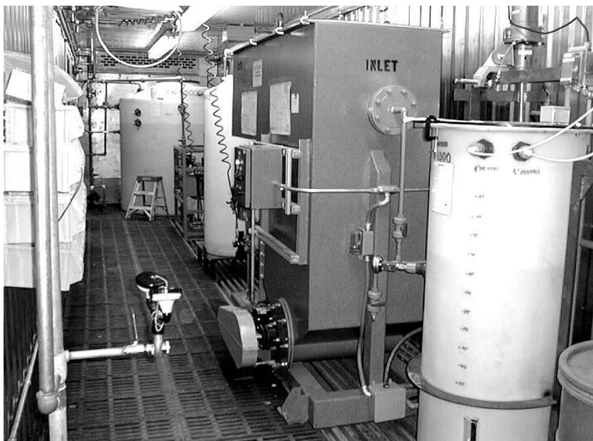
Figure 2. Fenton's reactor, clarifier, RO system, dirty water tank and recycle water storage tank in trailer two.
