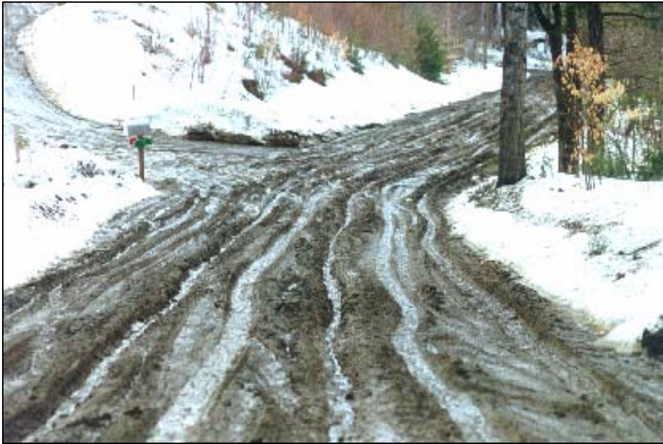
Figure 1. Rutting on unpaved secondary roads during spring thaw. (Photo by George Blaisdell, Hanover, NH.)
