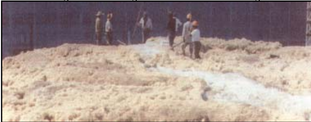
Figure 18 Constructing the Wet Storage Pile: Work Crew Directing the Flow
