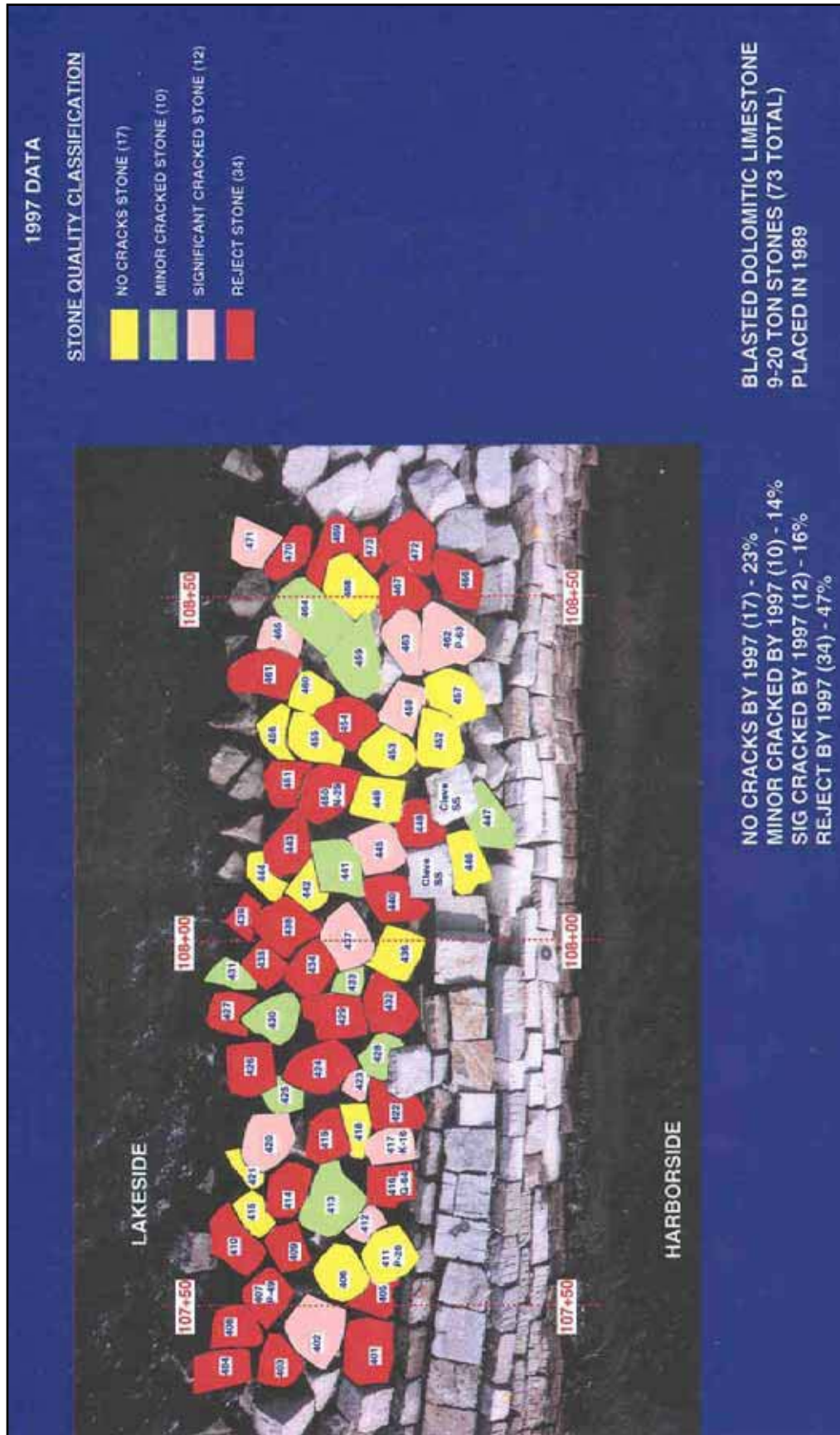
Figure 138. Cleveland Harbor east breakwater, sta 107+40 to sta 108+60, acceptable versus rejected stone, end of 1997
