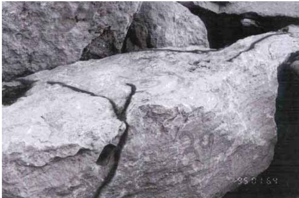
Figure 111. Significant cracks, Cleveland Harbor east breakwater, Marblehead Quarry low energy blasted dolomitic limestone, quality rating = 60 percent
