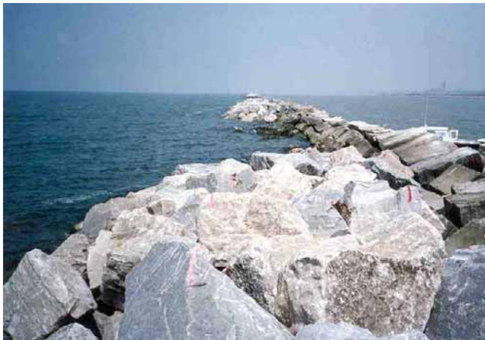
Figure 107. Cleveland Harbor east breakwater, Sandusky Quarry high energy blasted limestone (photo by Robert R. Bottin, ERDC)
