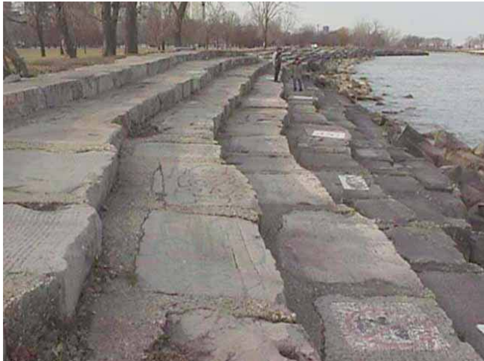
Figure A2. Limestone blocks in place along Chicago shoreline – Belmont to Diversey
