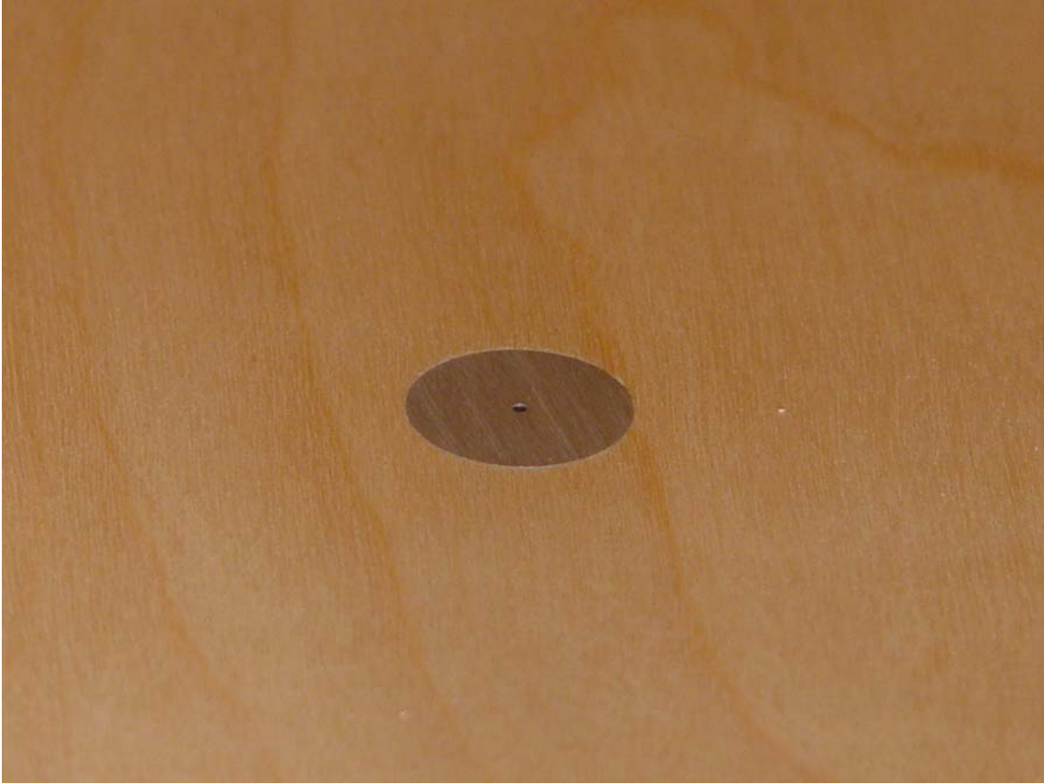
Figure 4.9. Oblique interior view of a static pressure port (note small opening in the center)
