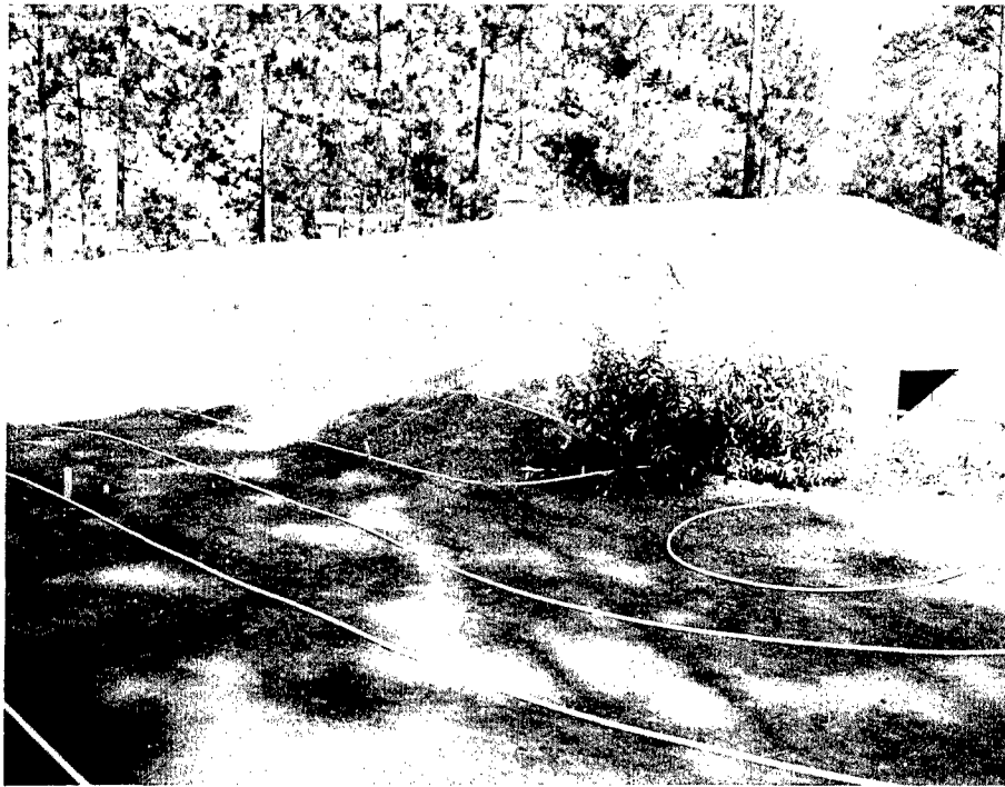
Fig. 2.13—Tubing layout at shelter.
