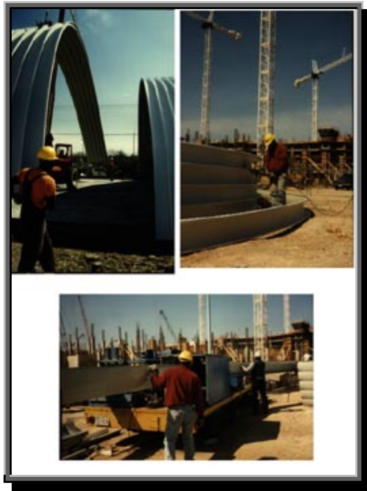
Figure 2.1. K-Span Construction (Spanco Building Systems, 2004:3)
