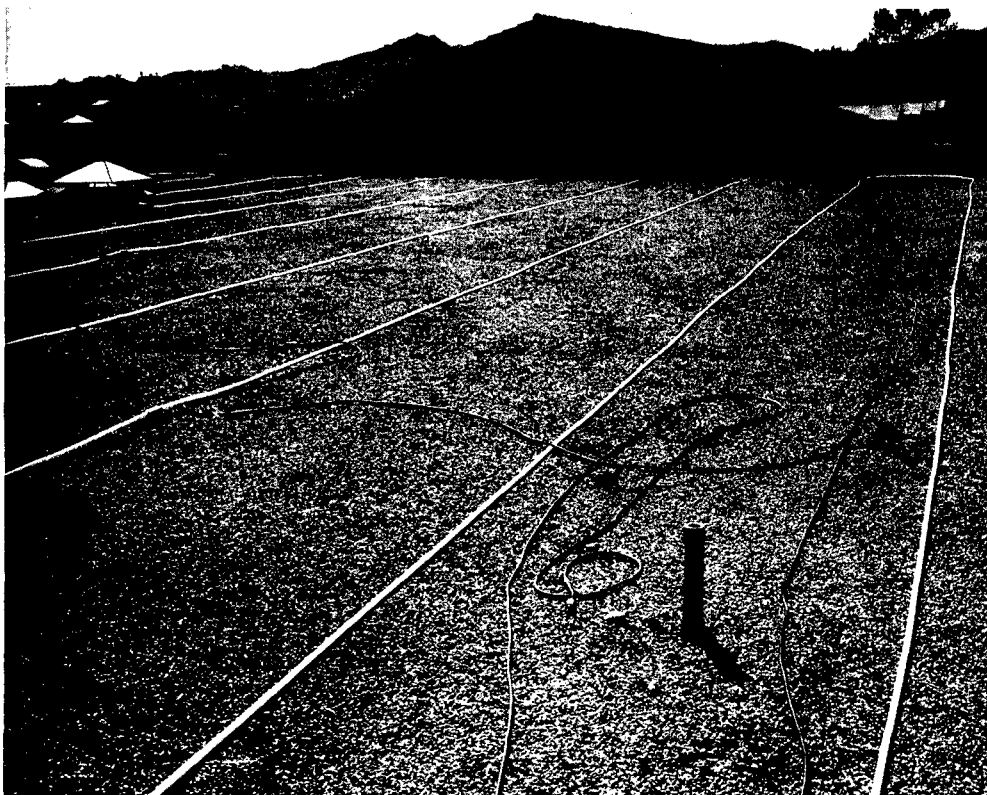
Fig. 2.25—Tubing placement on roof of North Hollywood High School classroom structure.
