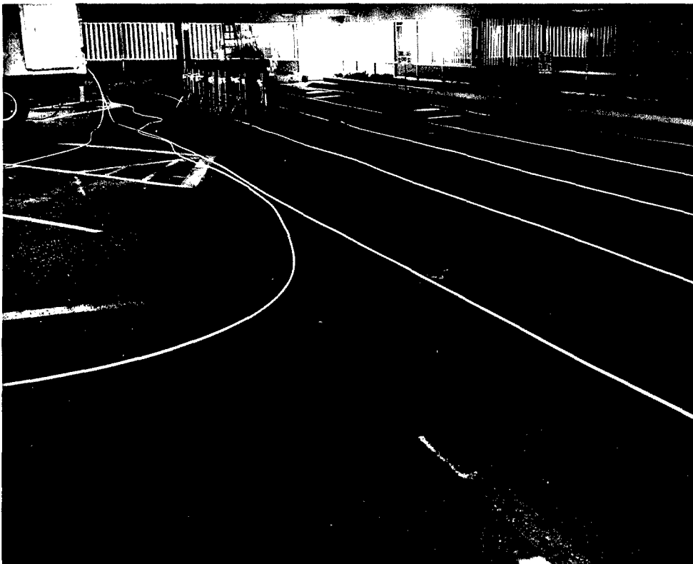
Fig. 2.24—Tubing placement on parking lot at Los Angeles Police Department building.
