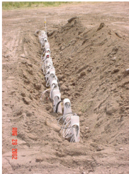
Figure 31. Top of risers prior to surface completion
