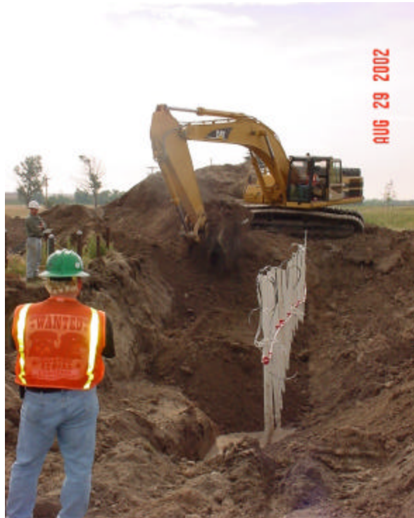
Figure 30. Backfilling of trench with imported soil. Note risers containing electrical connections, gas vests, washout tubing and multilevel sampling bundles
