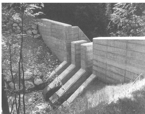
Figure 8. Stand-alone flow breakers (left) and flow breakers in debris dam (right) (from Fiebiger, 1997).
