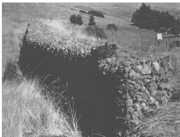
Figure 12. Gabion deflection wall, Tiburon, California (left), and design gabion deflection wall (right) (from Baldwin and others, 1987).
