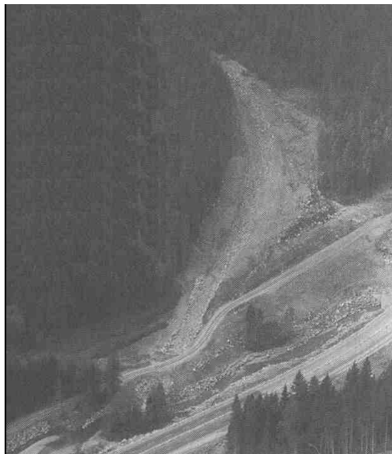
Figure 11. Deflection berm schematic (left) and deflection berm on Boulder Creek in British Columbia (right) (from VanDine, 1997).
