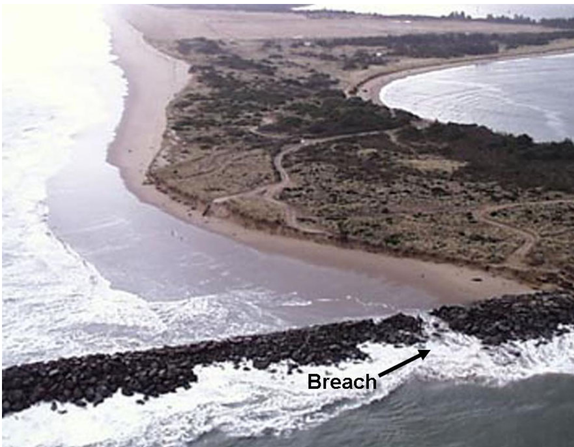
Figure 8. Coos Bay, OR, breach of north jetty (Hays et al. 2003)
