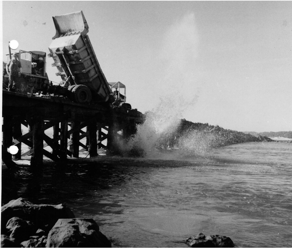
Figure 4. Rock fill by conventional end-dump method (Henshaw 1956)
