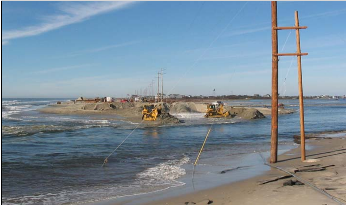
Figure 9. A view of first attempt to complete closure looking to west from eastern bank of breach (Wutkowski 2004)
