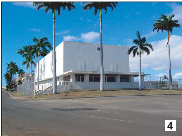
View looks at front of former theater from intersection of Hornet Avenue and Pokomoke Street, showing portico.
