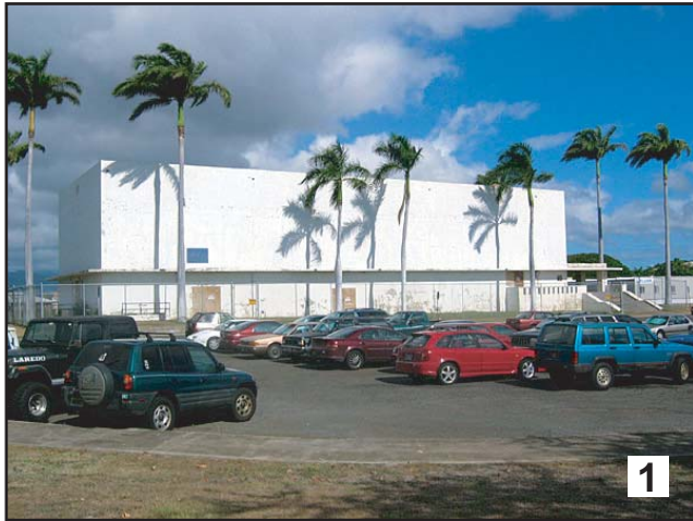
View looks from waterfront across existing parking lot and Hornet Avenue at east facade of Building 89.
