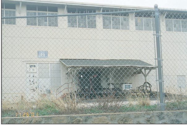
Loading platform addition at the middle of the south wall
