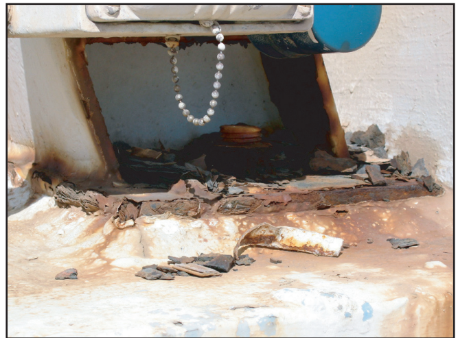
Close-up view of a rusted bolt holding a support beam of gantry crane tower to the lab concrete structure
