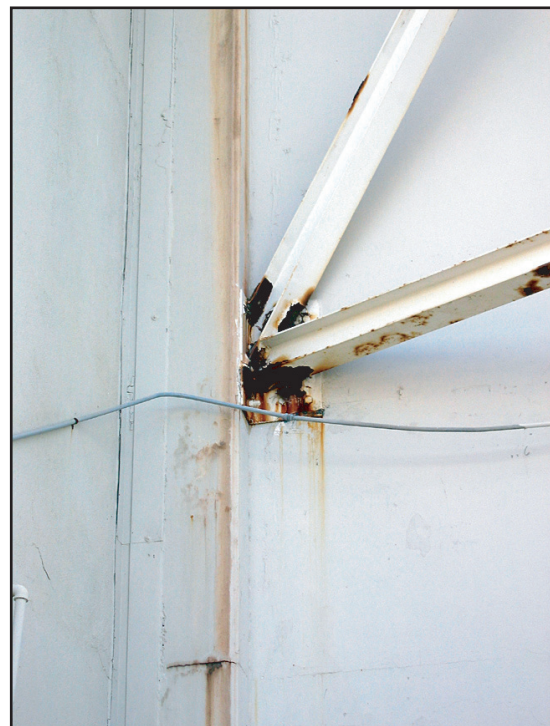
Close-up view of support beams bolted to the side of the lab concrete structure
