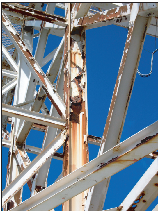
Close-up view of a (representative) rusted section of the gantry crane tower
