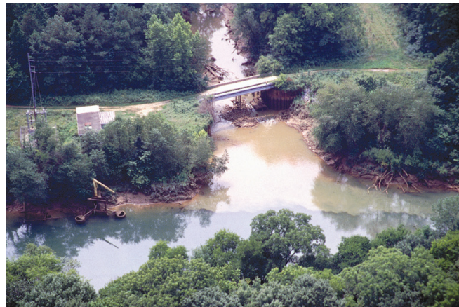
Sediment-laden runoff entering the Chattahoochee River from Suwanee Creek
