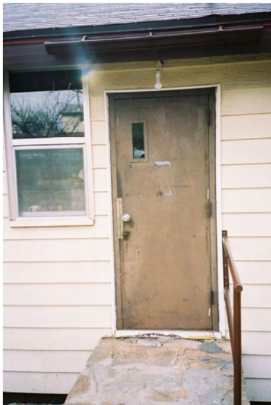
The metal gutter is above the northeast entrance door.
